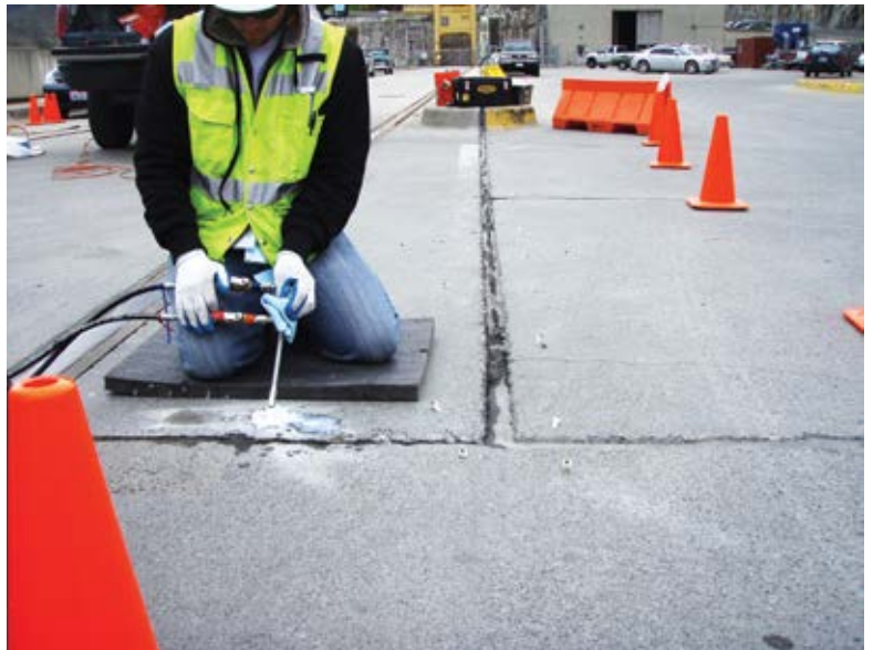
Fig. 10(b): MERL employee injecting grout
