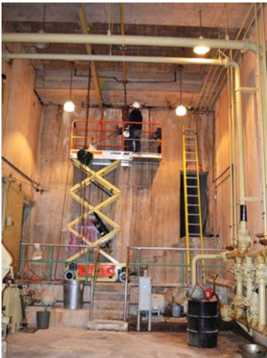
Fig. 3(b): Repairs being performed below transformer deck
