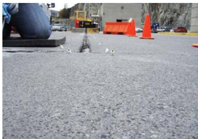
Fig. 2(b): Photo of grout ports and grease zerks
