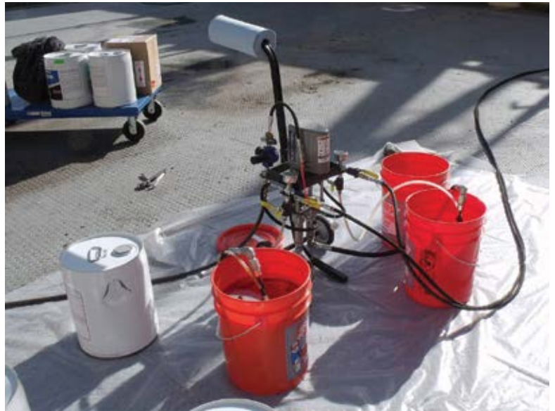
Fig. 9: Air-powered pump for grouting
