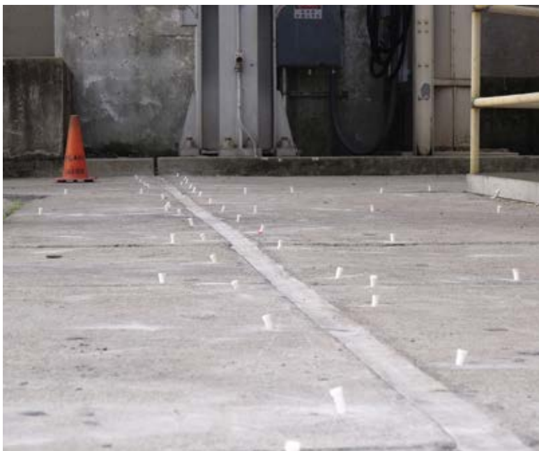
Fig. 8: Plastic ports for grout injection at Folsom Dam
