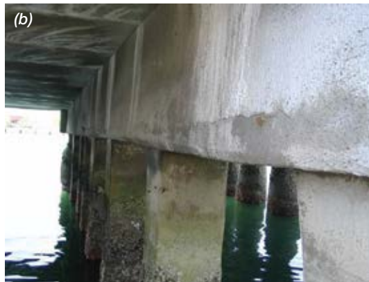
Fig. 8(a) and (b): Port of Canaveral—concrete deterioration prior to repair
