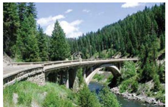
Fig. 6(c): Rainbow Bridge after repair
