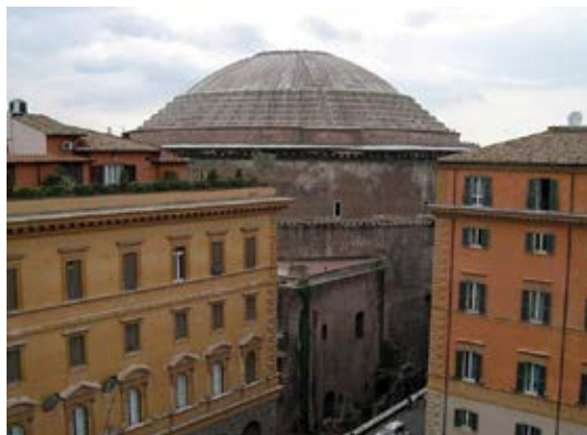
Fig. 2(b): Pantheon (Rome, Italy)—rear view (cast-in-place concrete dome)
