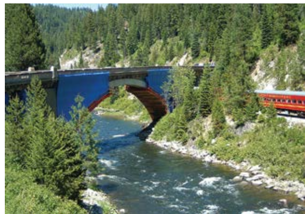
Fig. 6(b): Rainbow Bridge during repair and chloride extraction
