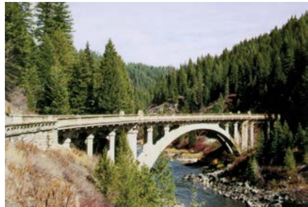
Fig. 6(a): Rainbow Bridge before repair
