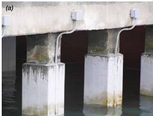
Fig. 8(a) and (b): Port of Canaveral—concrete deterioration prior to repair
