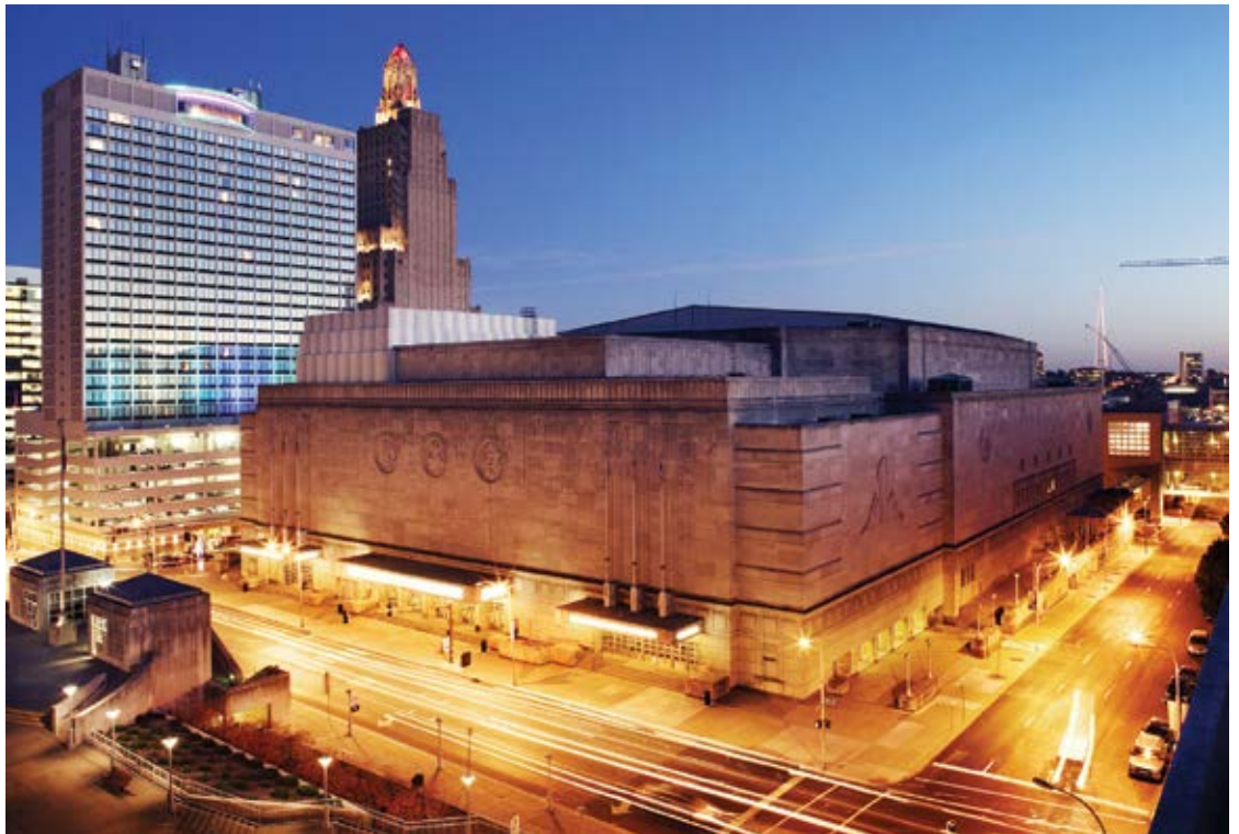
Fig. 1: Kansas City Municipal Auditorium, circa 2012 (Image courtesy of the Kansas City Convention & Visitors Association)
