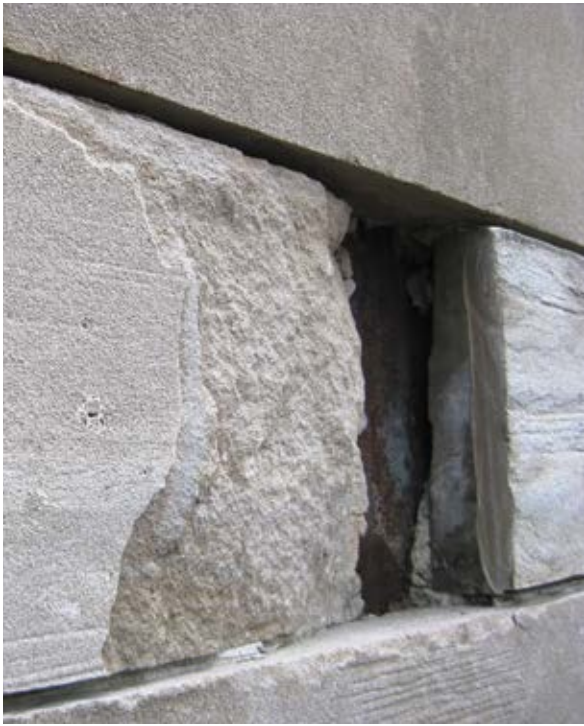
Fig. 4: Corrosion of a structural steel column that resulted in damage to the stone veneer. Note that steel is directly behind with veneer with no protection from moisture
