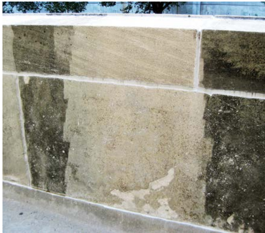
Fig. 5: Successful cleaning mockup, showing level of heavy soiling removed
