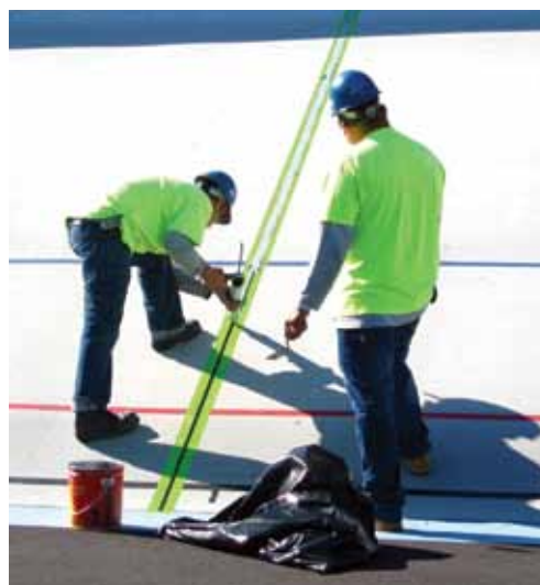
Installation of traffic grade sealant for repair of a transverse joint
