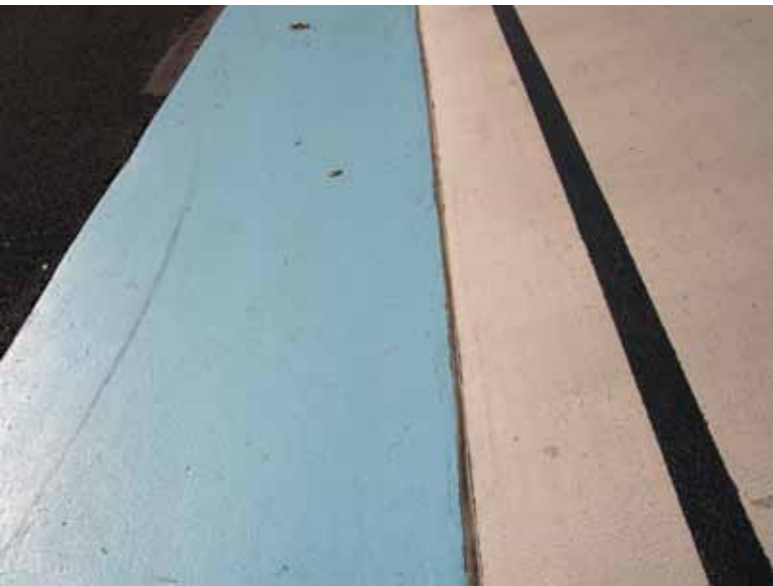
Repaired inside perimeter joint
