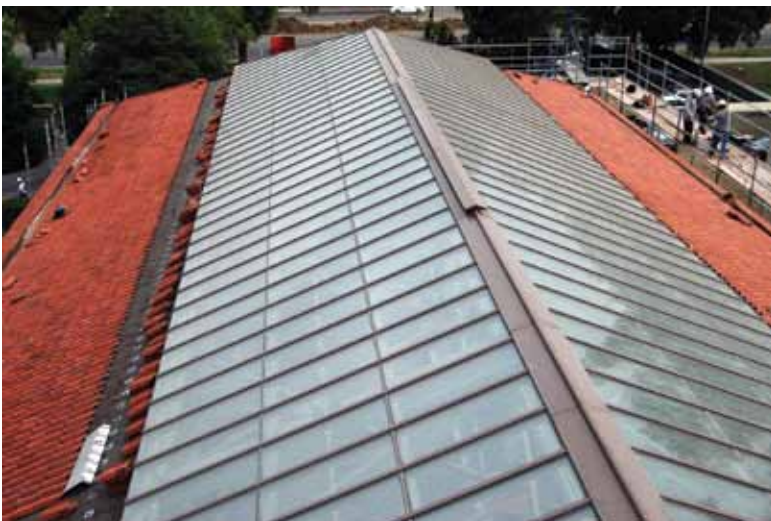
Fig. 8: Restored shingles replaced on the roof with new skylights
