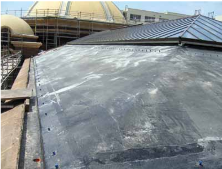
Fig. 7: Retrofitted slab after broadcasting of sand on top of CFRP
