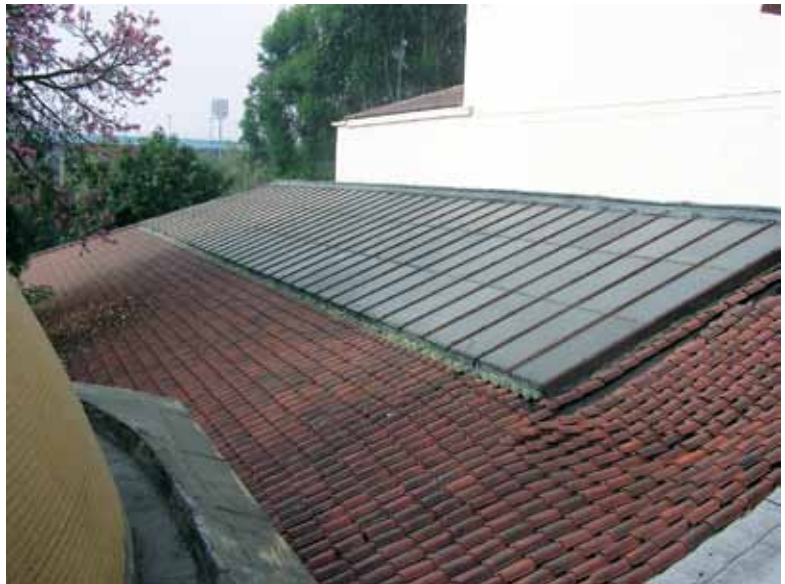
Fig. 3: View of roof and shingles before seismic upgrade
