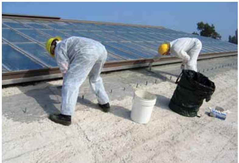
Fig. 4: Smoothing the rough concrete deck
