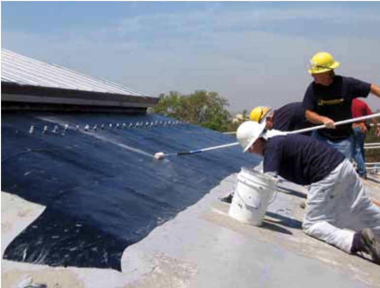
Fig. 6: Installation of CFRP strips over protected steel bolts
