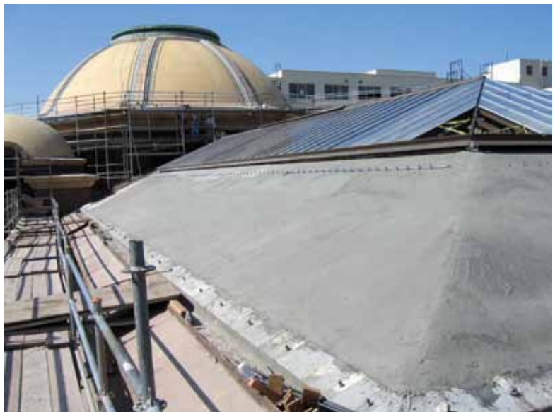
Fig. 5: Roof deck after it has been prepared for CFRP installation
