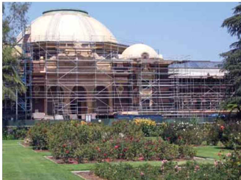
Fig. 2: Building with scaffolding during seismic upgrade in summer 2007
