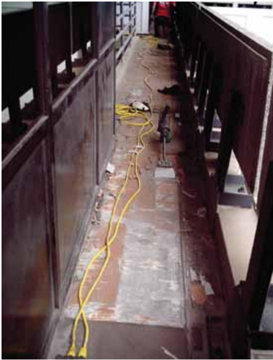
Fig. 3: Concrete surface preparation on walkways
