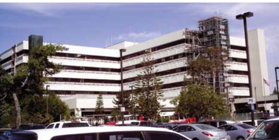
Fig. 2: View of walkways
