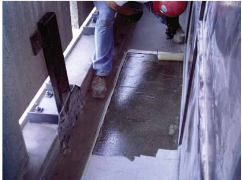
Fig. 4: Application of primer coat to walkways
