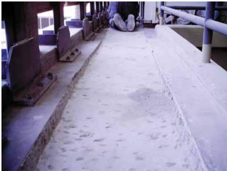
Fig. 7: Milled-down surface of walkways
