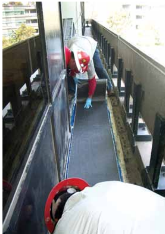
Fig. 5: Carbon-fiber fabric being applied to walkways
