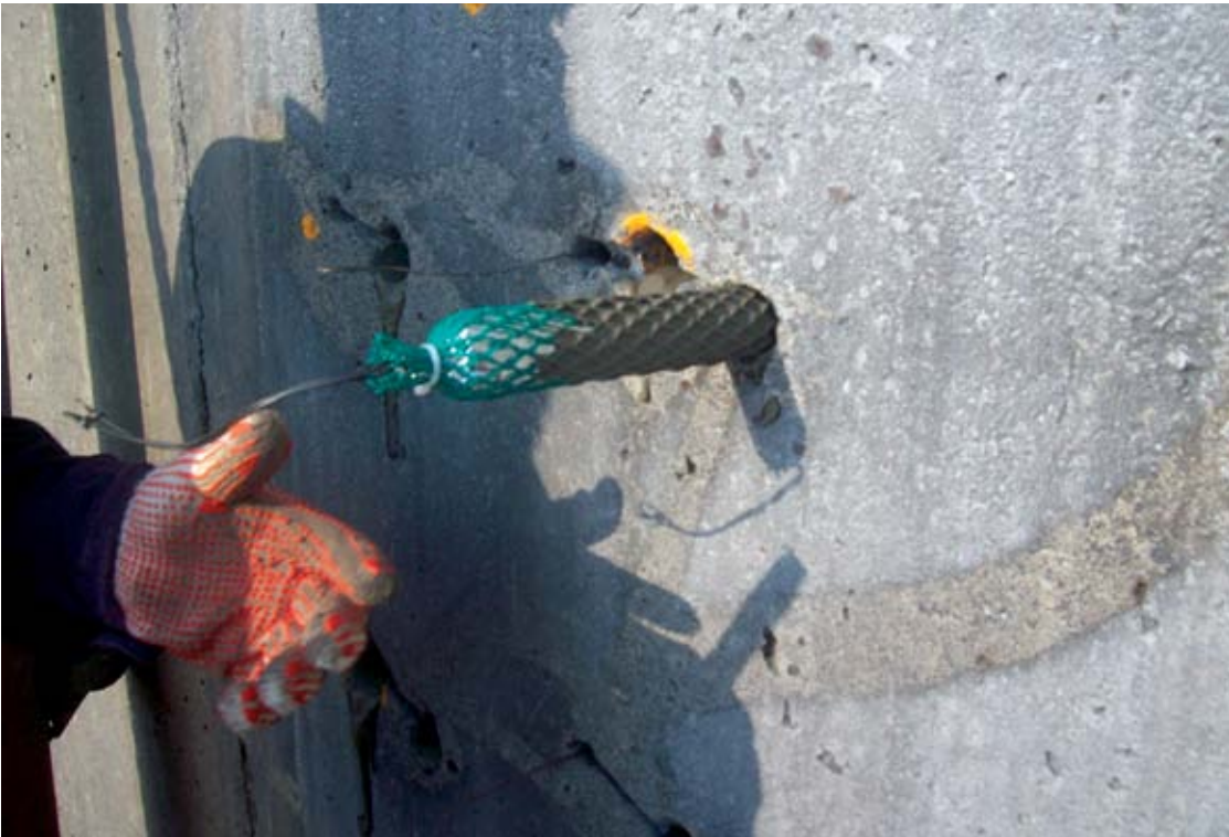
Fig. 7: Installation of zinc anodes
