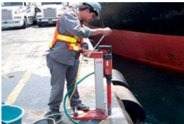
Fig. 4: Concrete core removal
