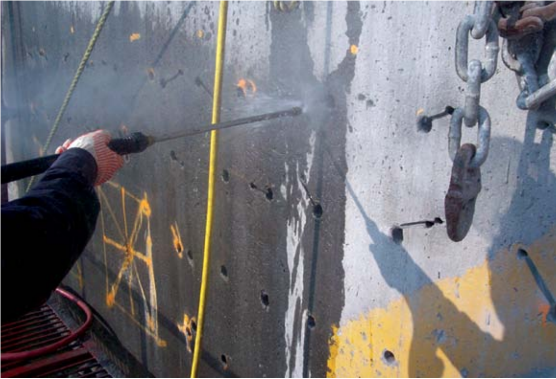
Fig. 6: Removing and cleaning concrete
