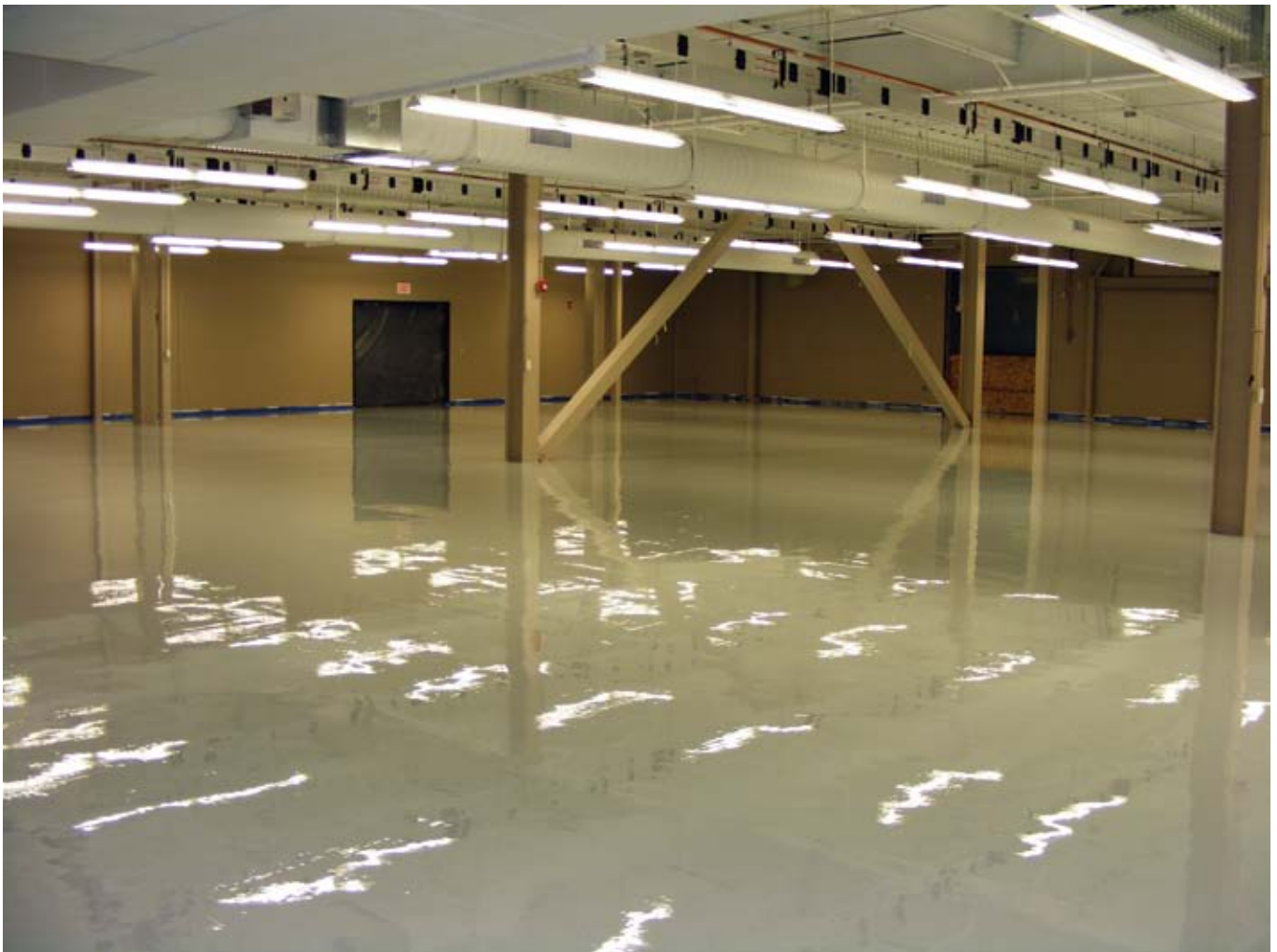
Garmin's ESD floor after completion of installation
