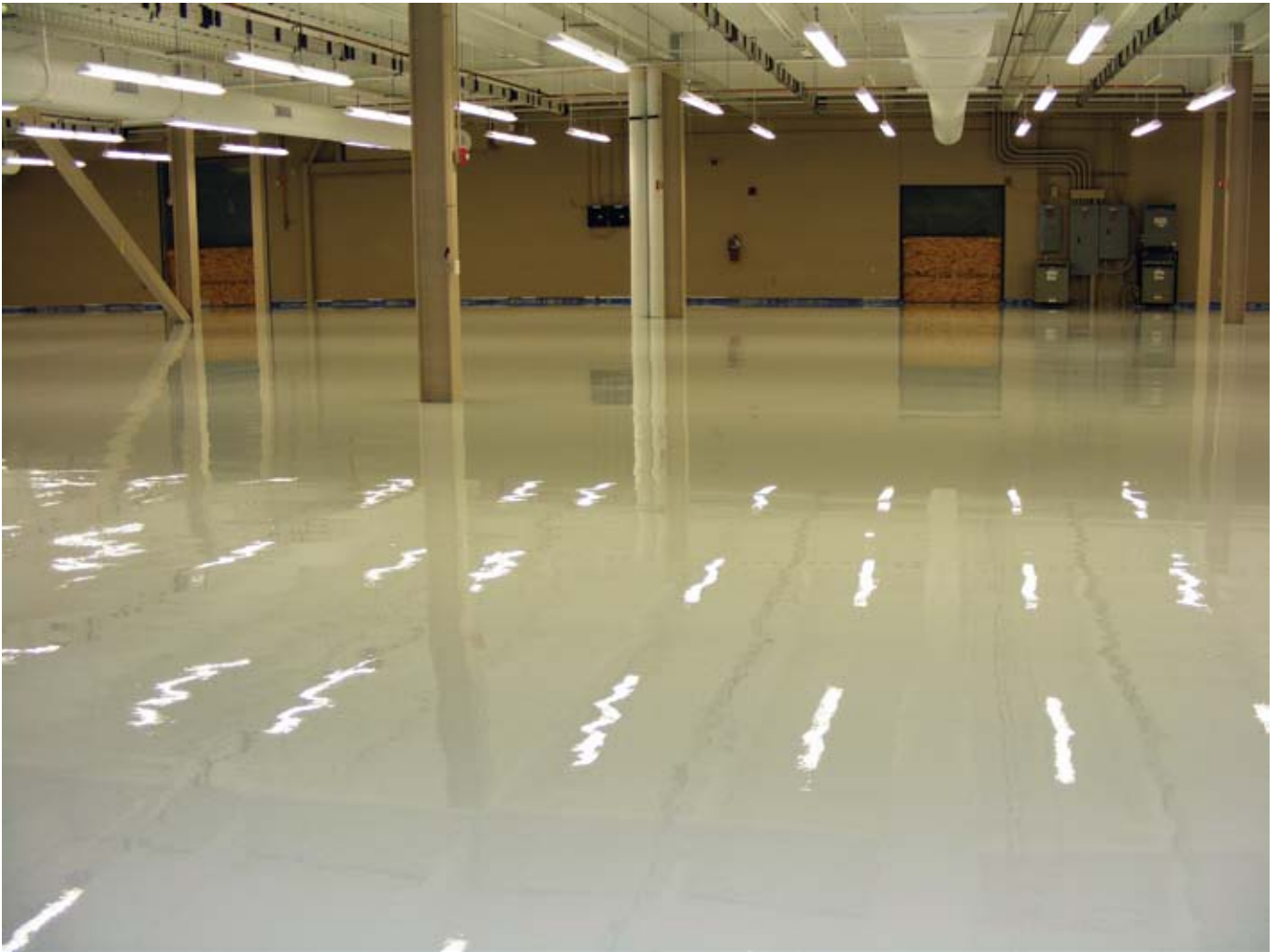
Garmin's ESD floor after completion of installation
