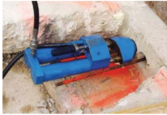
Fig. 9: Strands are stressed using a monostrand ram
