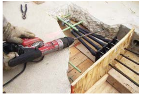
Fig. 5: Installation of reinforcement for anchorage pocket
