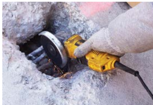
Fig. 2: PT strands are cut using a grinder
