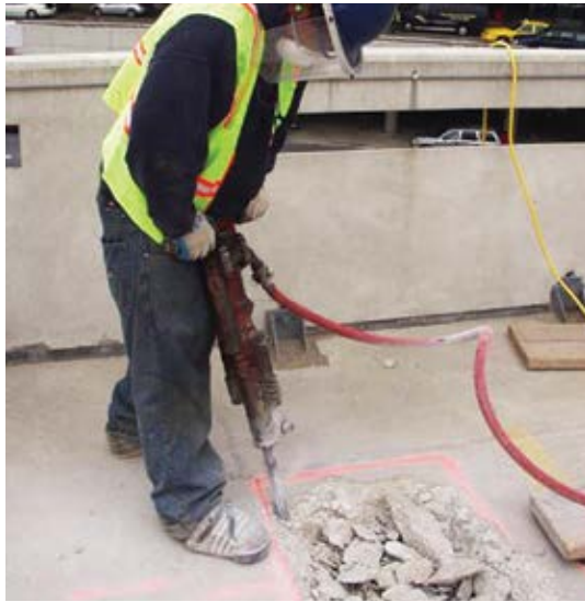
Fig. 3: Anchorage pockets being chipped out
