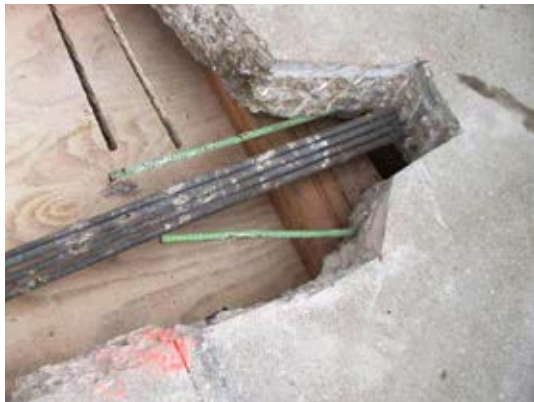
Fig. 4: Anchorage pocket after chipping
