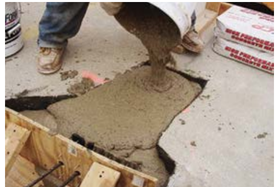
Fig. 7: Pouring anchorage pocket
