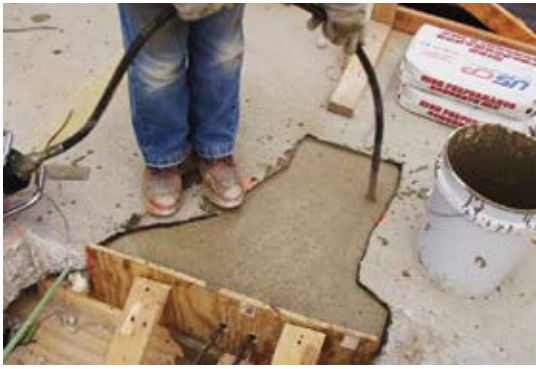
Fig. 8: Vibrating repair material for proper consolidation
