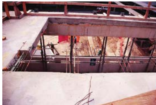
Fig. 10: Excess concrete is removed from the new opening
