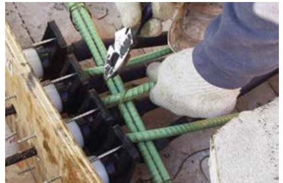
Fig. 6: Tying steel at anchorage point
