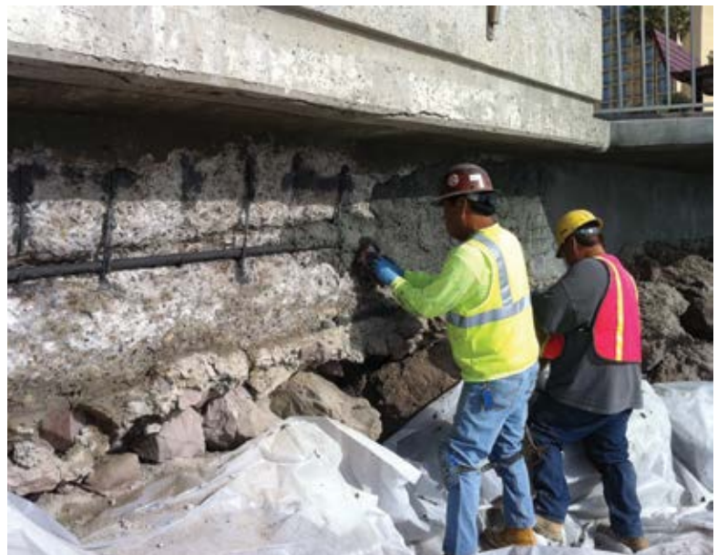
Fig. 7: Patching grade beam wall
