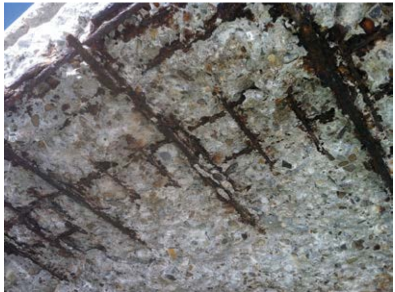
Fig. 6: Condition after initial demolition
