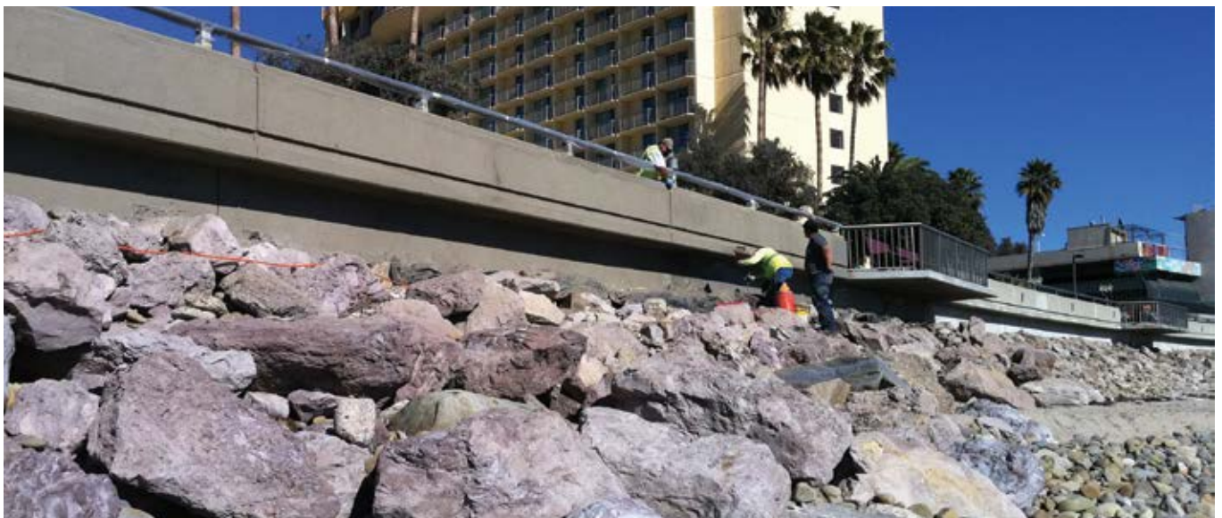
Fig. 11: Applying final finish
