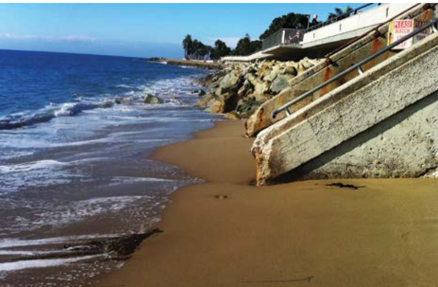
Fig. 1: Ventura seawall coastline
