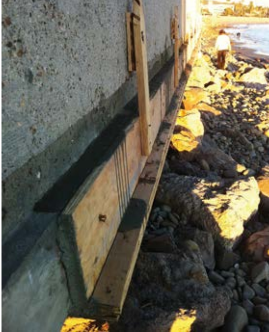
Fig. 8: Forms in place
