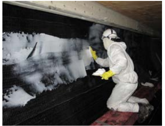
Fig. 11: Application of saturation epoxy
