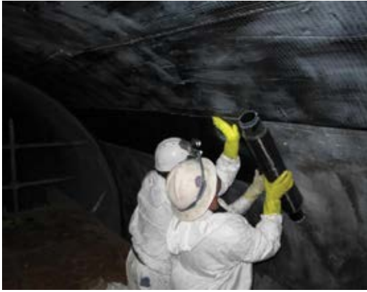
Fig. 8: Longitudinal application of fabric
