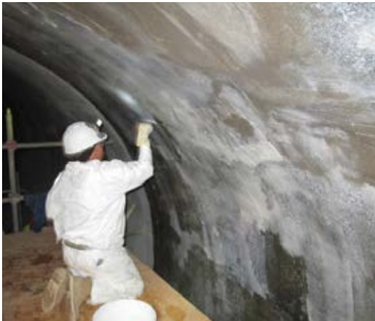
Fig. 5: Application of saturation epoxy
