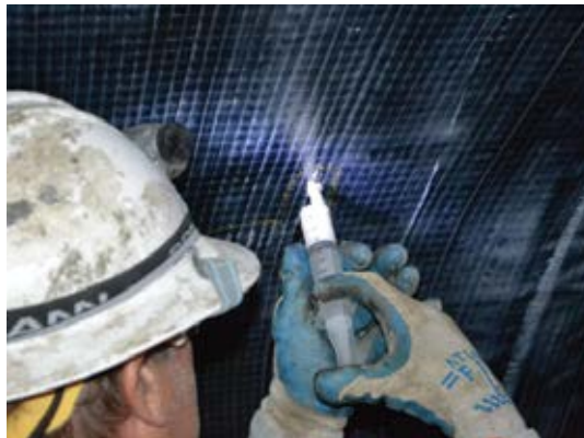
Fig. 14: Epoxy being injected
