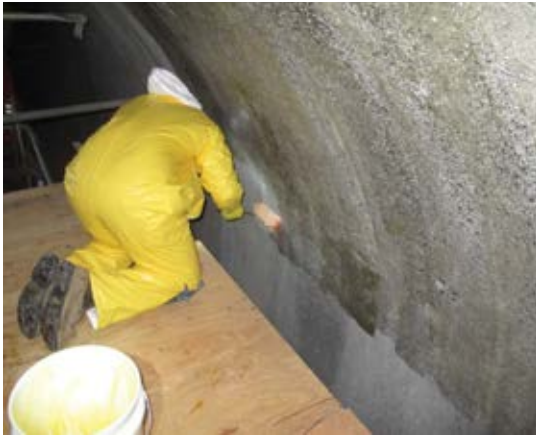
Fig. 4: Application of epoxy primer
