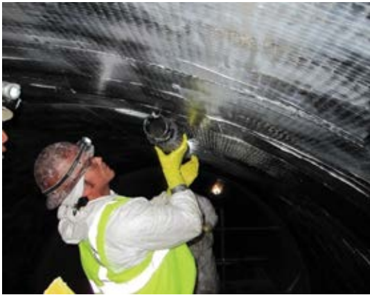
Fig. 9: Applying fabric in hoop direction
