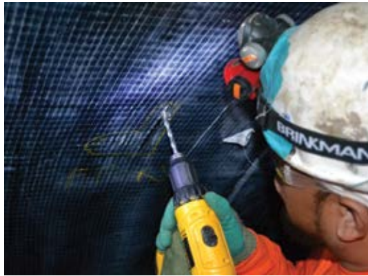
Fig. 13: Hole being drilled for epoxy injection
