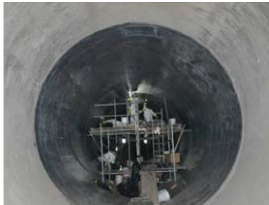
Fig. 1: Completed CFRP-lined section
