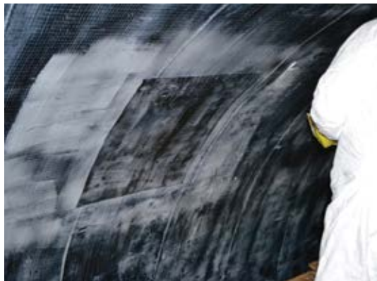
Fig. 16: Patch repair of delaminated area
