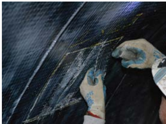
Fig. 15: Cutting out delaminated layers
