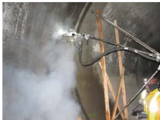
Fig. 2: High-pressure hydroblasting
