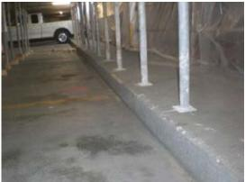
Fig. 1: Temporary shoring and dust control measures
