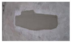
Fig. 13: Final surface of patch repair
