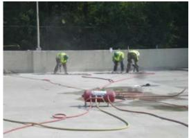
Fig. 2: Workers exposing tendons with small chipping hammers
