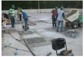
Fig. 12: Consolidating patch material
