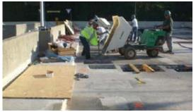
Fig. 11: Pouring concrete repair material
