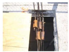
Fig. 6: Spliced cables
