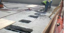
Fig. 3: Exposed anchor locations
