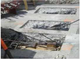
Fig. 7: Spliced cables ready for tensioning
