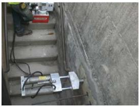
Fig. 8: Tensioning new cables in stairwell
