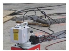
Fig. 9: Tensioning new cables on deck
