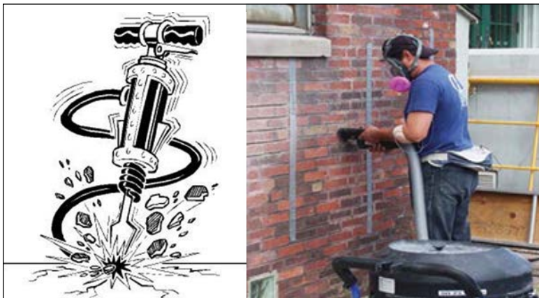
Fig. 1: Jackhammer and grinding equipment
