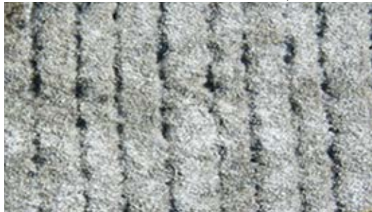
Fig. 6: Typical application at the Grand Ronde River Bridge in Oregon
