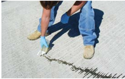
Flood surface with properly mixed epoxy
