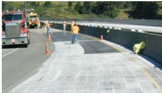
When cured, remove excess sand and open to traffic
