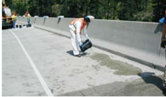
Use rollers or squeegees to distribute resin material
