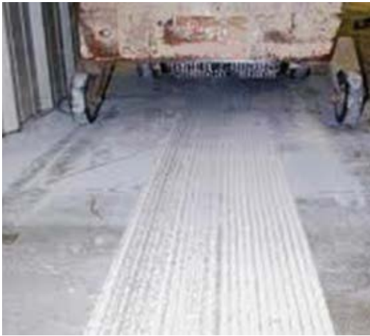
Fig. 5: Concrete removed during scarification
