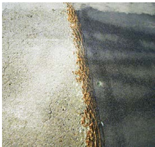
Fig. 4: Surface preparation to remove coating
