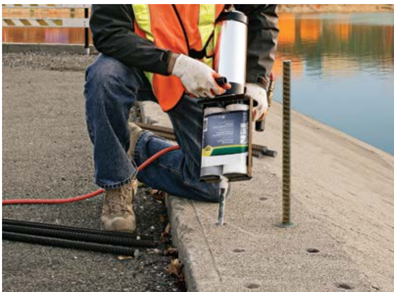
Fig. 1: Installing new reinforcing bars into existing concrete using adhesive
