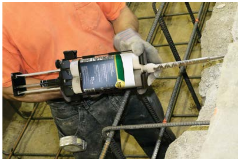
Fig. 2: Side-by-side dual cartridge adhesive product with static mixing nozzle
