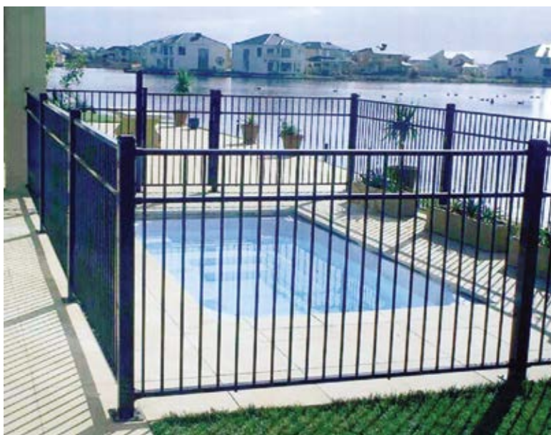
Fig. 5: Repair to pool decks can result in requirements for providing new gates or barriers (Photo attributed to A-Confence Pty Ltd)
