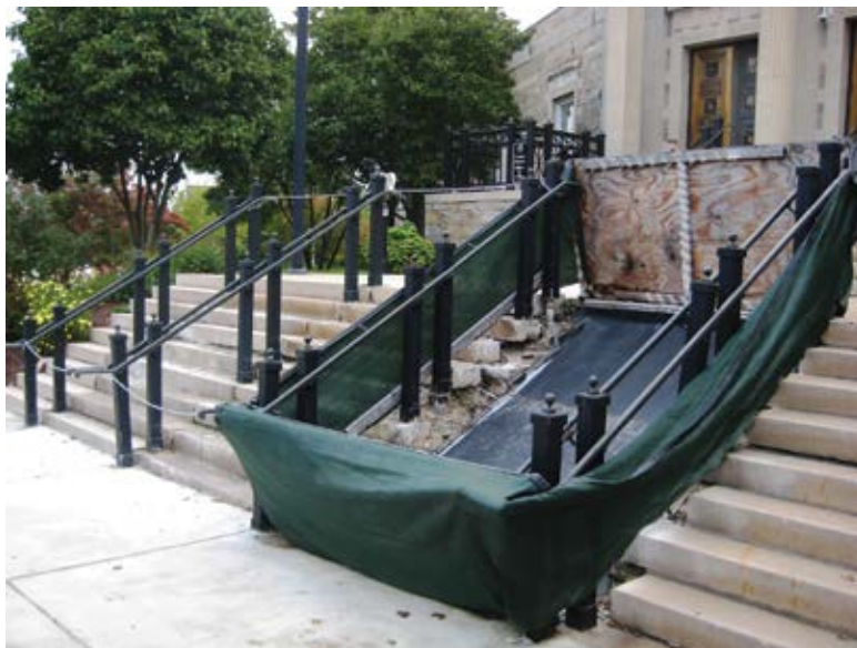
Fig. 4: Step repair at government building
