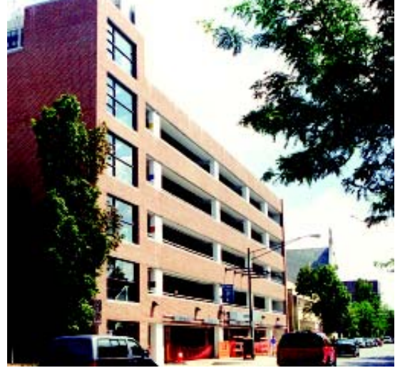
Renovation complete—Thompson Street view
