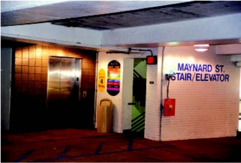
New elevator/stair area with new signage
