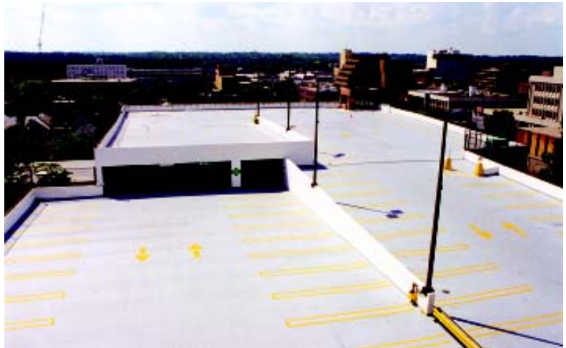
Completed rooftop deckcoating
