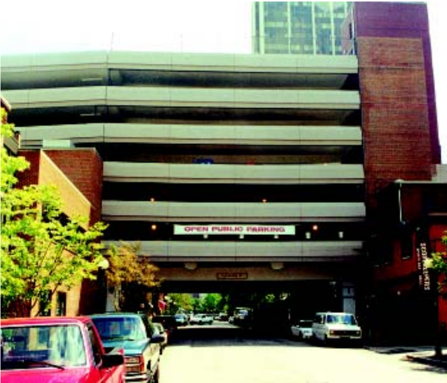
Renovated structure—Maynard Street view
