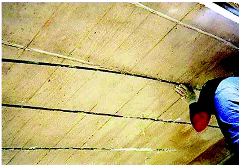
(a) Installing CFRP rods
