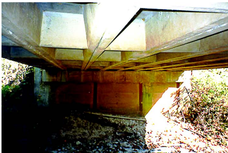
Figure 6: The underside of Coats Lane Bridge
