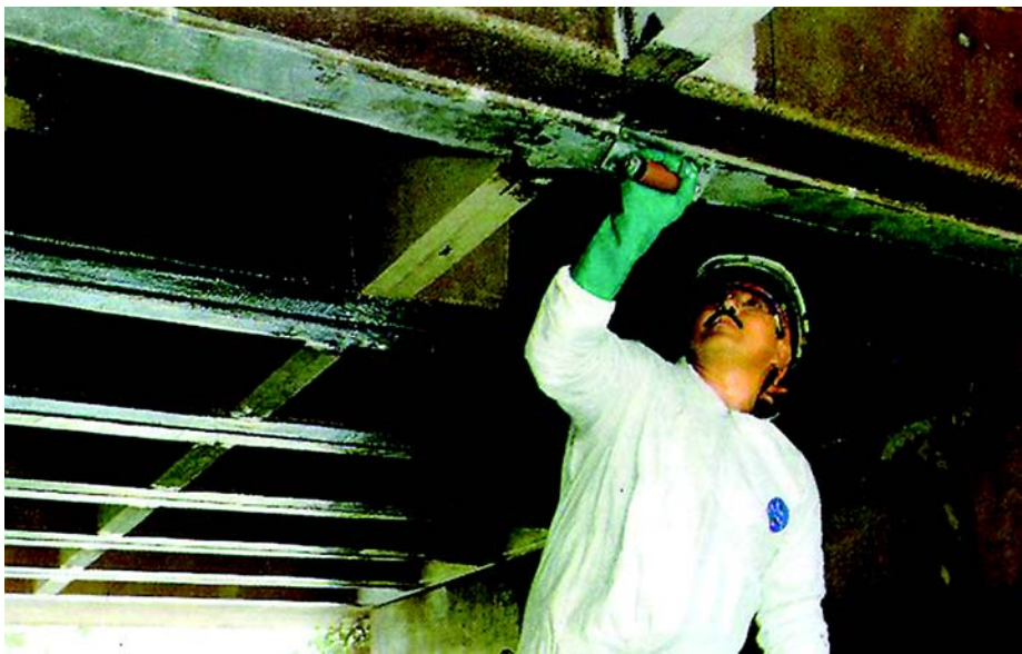
Figure 8: Application of CFRP strengthening
