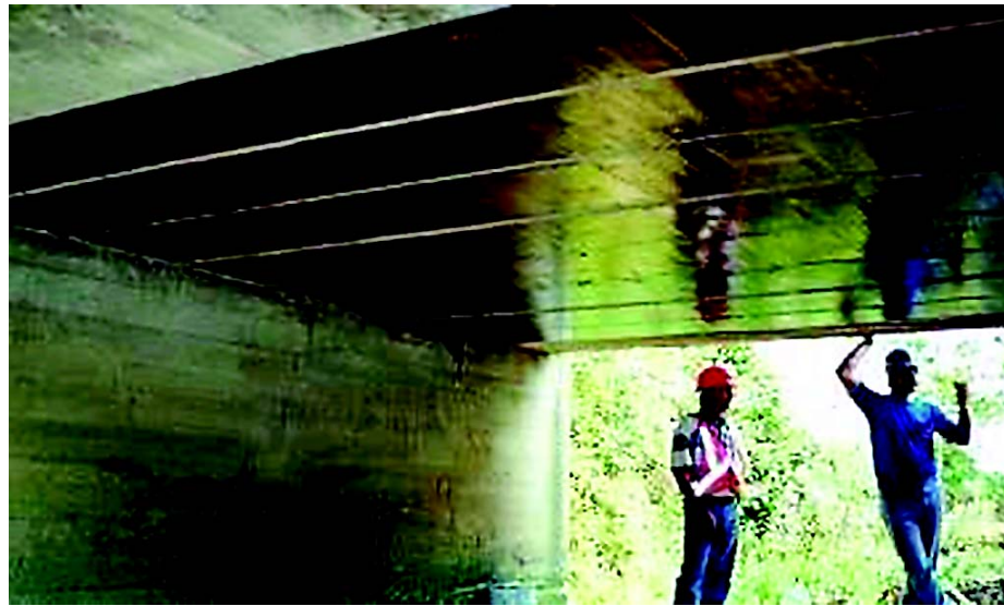
Figure 2: CFRP reinforcement bonded to the underside of Bridge G270
