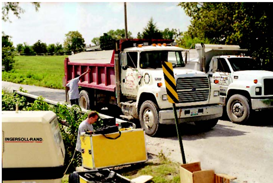
Figure 10: Bridge in-situ load testing
