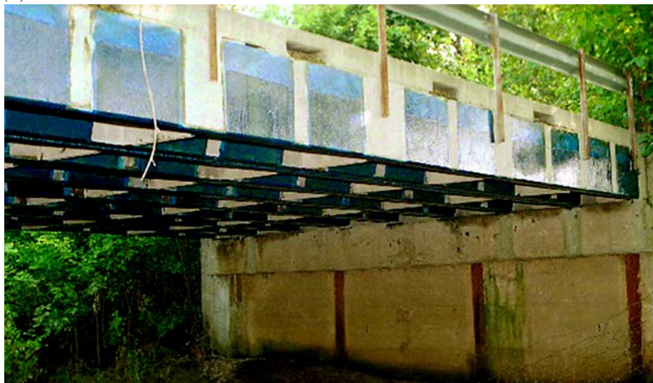
Figure 9: Coats Lane Bridge before (a) and after (b) strengthening
