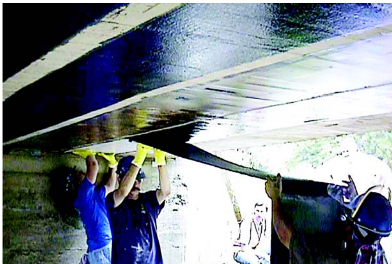
(b) Installing CFRP sheets
