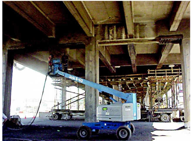
Shooting in progress on crossbeam
