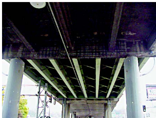
Underside of bridge prior to shooting
