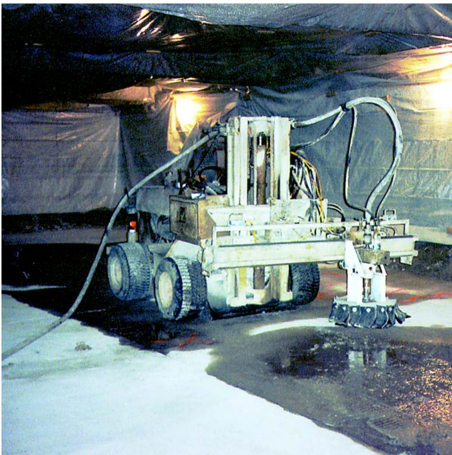
Remote-controlled Hydrodemolition Robot
