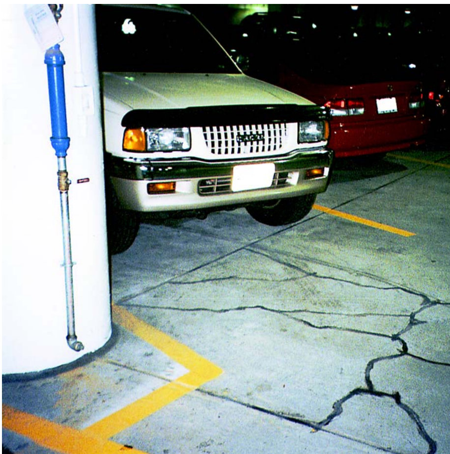
Column area after concrete repair
