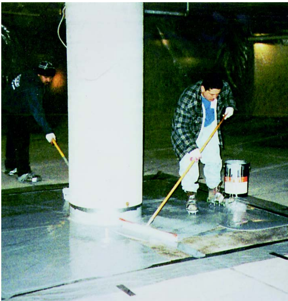
Column area after concrete repair receiving coating
