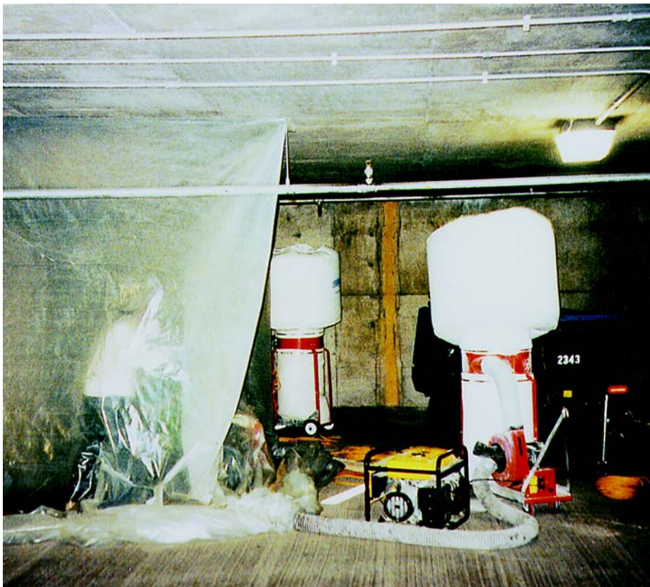
Shotblasting of column area inside containment before receiving coating
