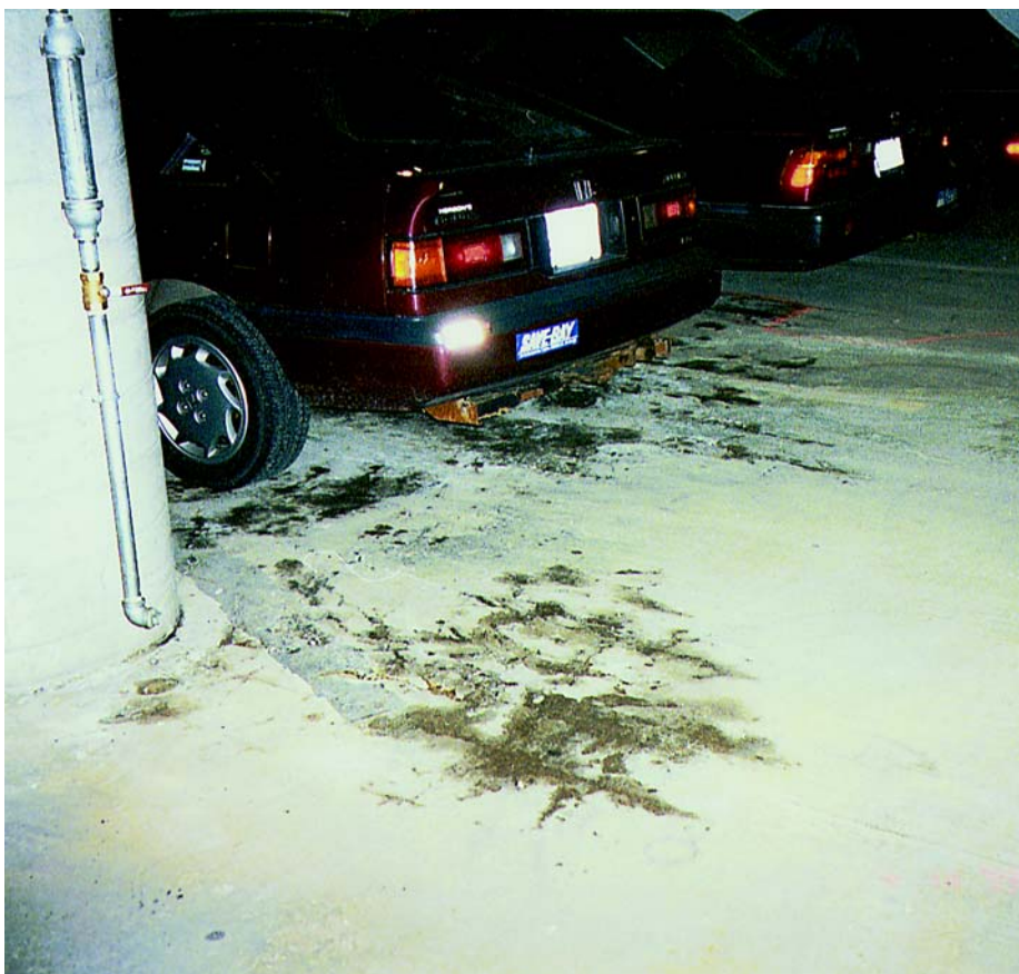
Column area before concrete spall repair
