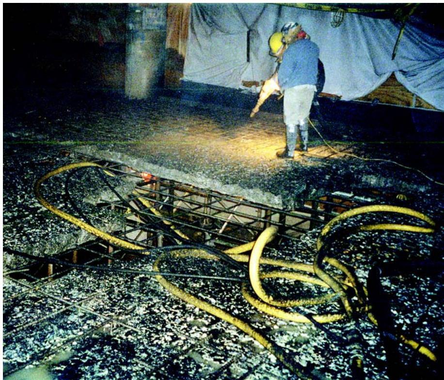
Cleaning of steel after hydrodemolition
