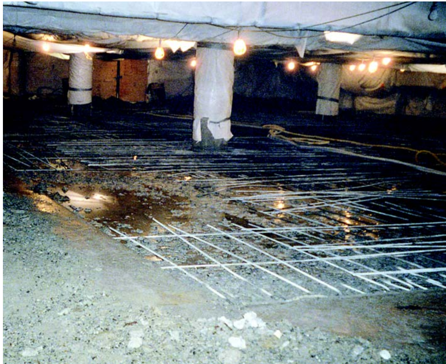
Exposed top steel after hydrodemolition
