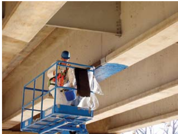
Application of second fiber sheet
