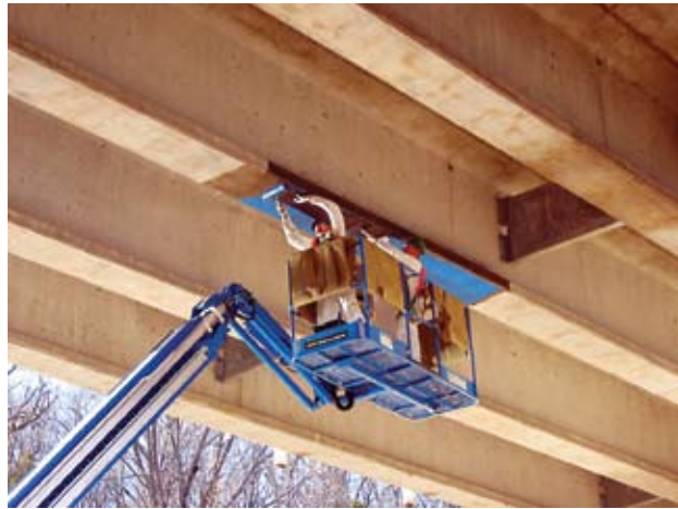
Application of first fiber sheet
