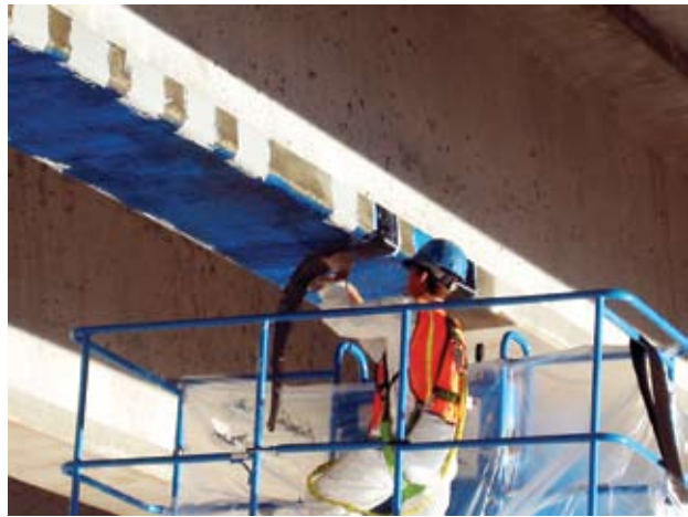
Application of U-wraps
