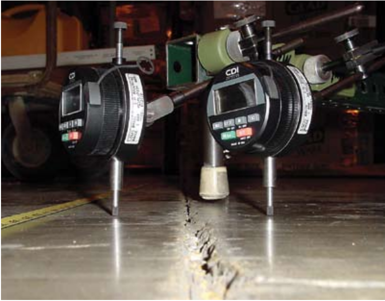
Fig. 5: A Modified Benkelman Beam is used to determine joint stability and load-carrying capacity of the slab
