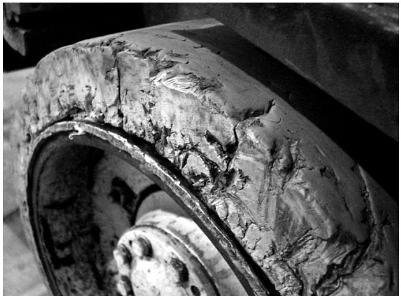
Fig. 3: Lift truck tire damage due to widespread joint spalling
