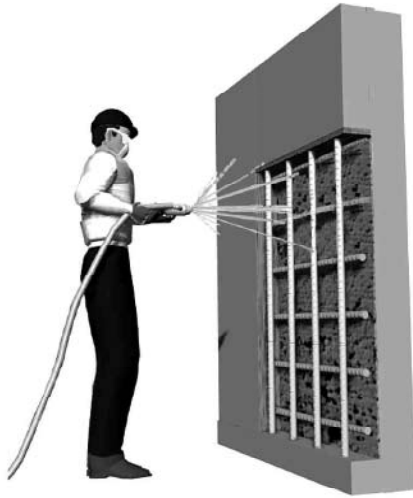
Fig. 3—Presaturate prepared surface with water.
