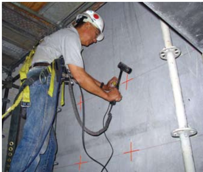
Impulse-Response testing on the inside surface of the panel
