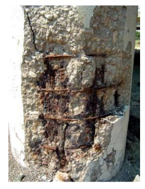
Work began in August of 2003 after the support system for handling the heavy loads had been designed and fabricated. In areas were there was a significant section loss, the pier cap had to be shored while under traffic. The support system put in place had to be able to withstand live loads of one of the busiest interstates in the state. The contractor worked closely with TxDOT and its consulting engineer to create the best shoring system possible.
