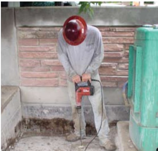
Drilling of injection ports
