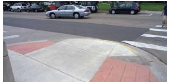
Ramps at Euclid Autopark
