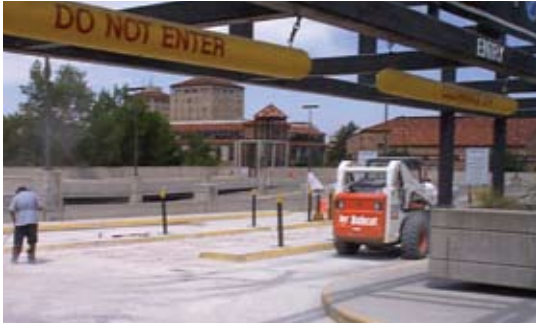
Slab prepared for deck coating
