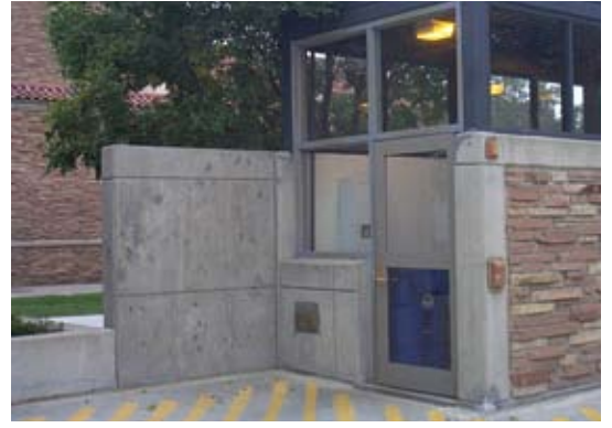
Interior face of wind wall
