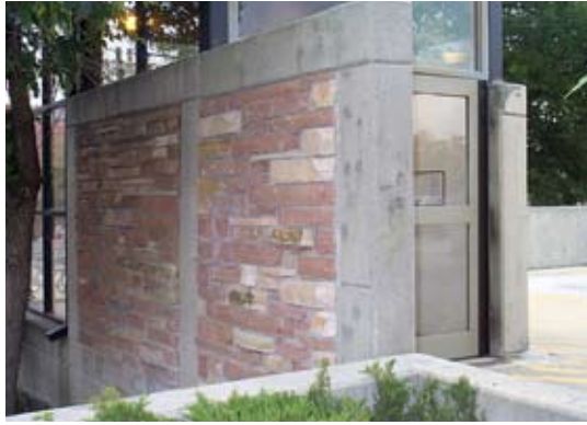
Exterior face and corner
