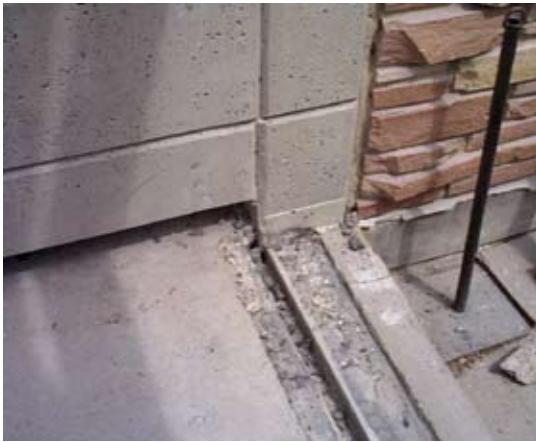
Expansion joint preparation
