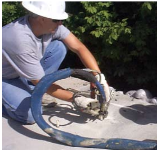
Pressure injection of grout
