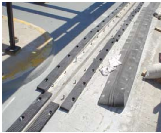
Expansion joint installation
