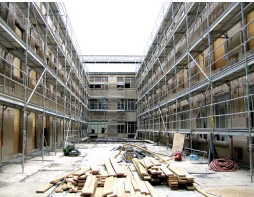
Fig. 2: Scaffolding constructed to allow direct access to walls
