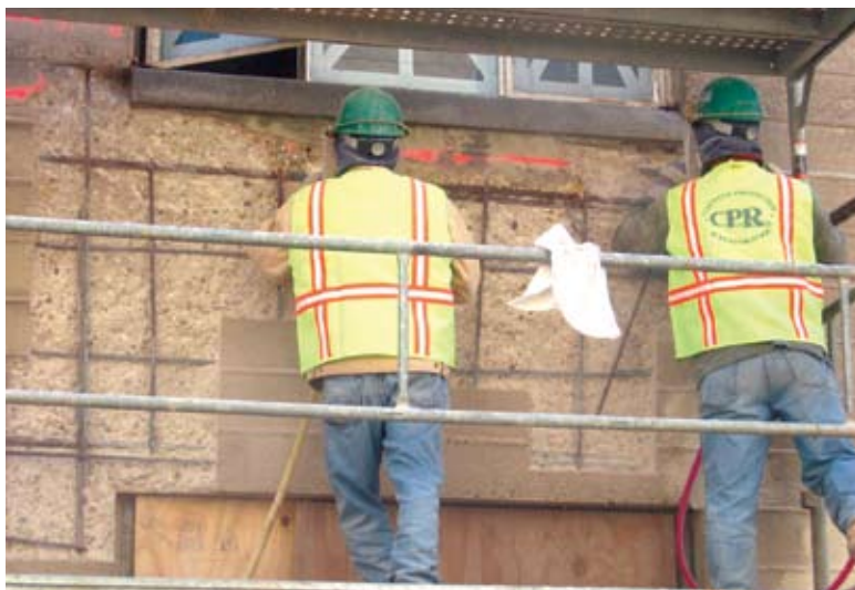
Fig. 3: Jackhammer demolition in progress, exposing corrosion-damaged reinforcing bars
