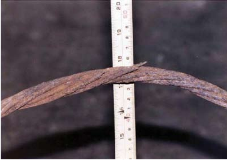
Failed strand from post-tensioned tendon
