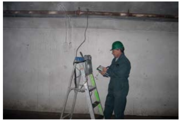
Taking readings for the PT corrosion evaluation
