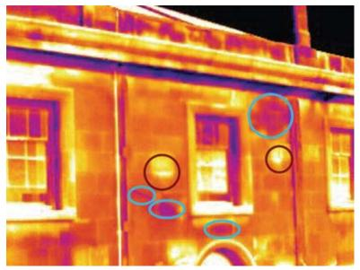
*Fig. 5: Thermography output showing areas of moisture retention, circled in blue, and previous spalls and repairs, circled in brown*
