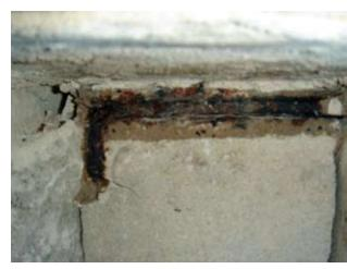
Fig. 7: Iron cramp exposed during preview to show condition; this agreed with a position that was deemed high risk by the condition survey. Note the end of the dog cramp to the left shows the emergence of a crack developing from the tip
