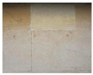
Fig. 2: Aesthetic deterioration caused by the unsightliness of cracking of the stonework. Note the crack developing from a previous repair where all the iron was not removed
