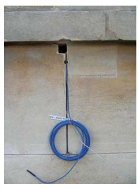
Fig. 10: Position showing discrete breakout for drill and tap steel connections and reference electrode monitoring installation
