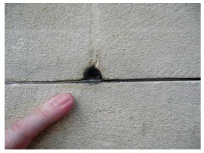
*Fig. 9: Anode drilled and grouted into position with interconnection wire ready for retucking*
