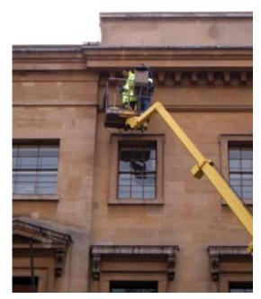
Fig. 4: Accessing from the street for surveying
