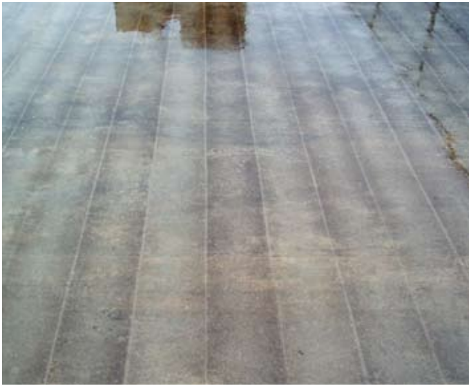
Concrete surface after shotblasting
