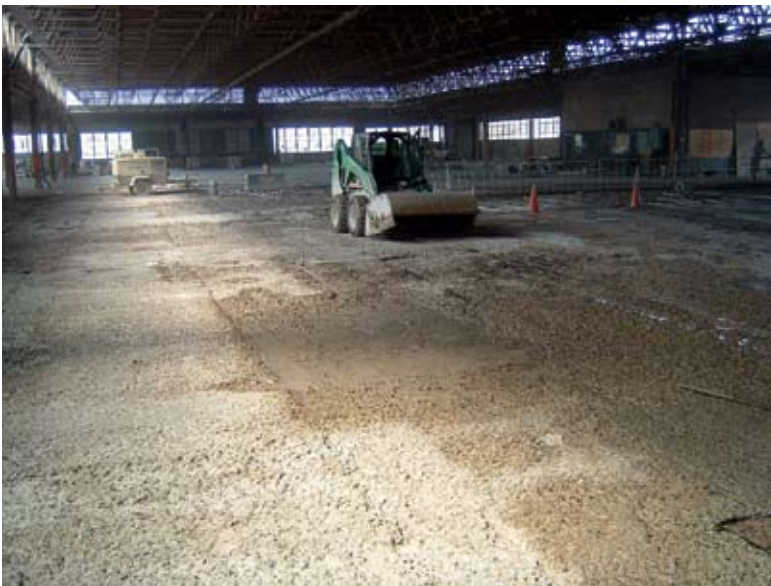
Deck after hydrodemolition
