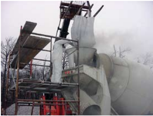
Mixing super sacks into concrete trucks
