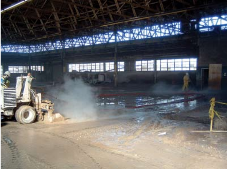
Hydrodemolition of deck
