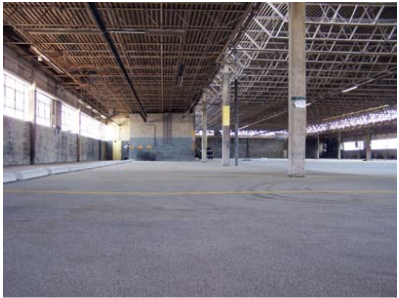
Bus terminal repair completed
