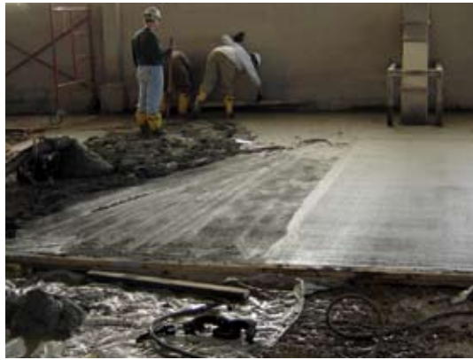
Placing pumped concrete
