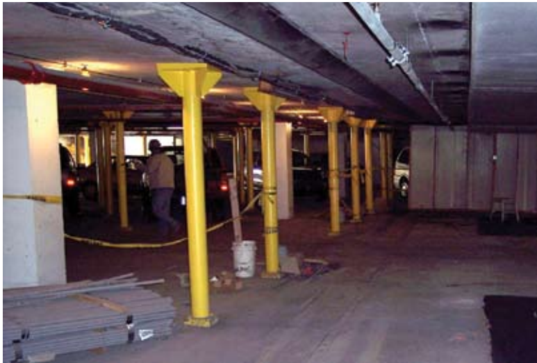
Repair project with shoring in place
