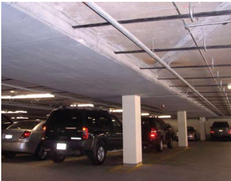
Completed parking bay
