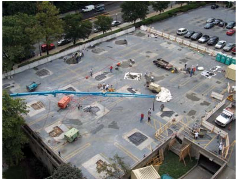
Top deck of garage during repairs
