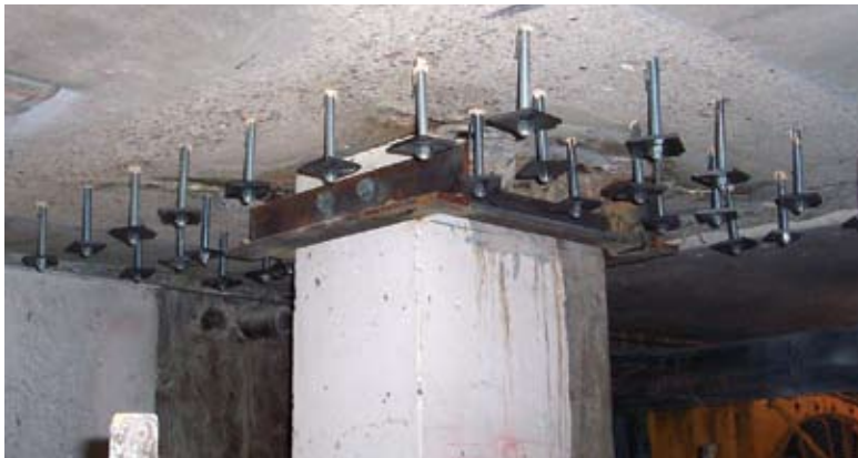
Typical repair around columns
