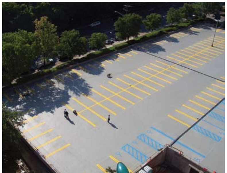
Top deck of garage after all repairs, deck coating, and striping
