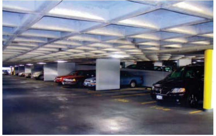
A finished interior with new striping and wheel stops
