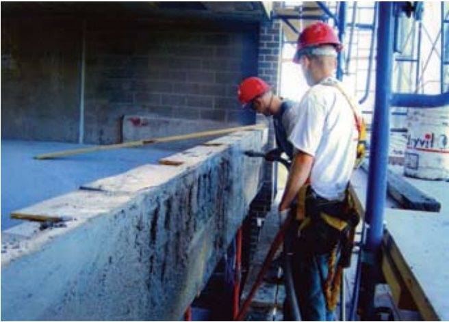
Façade work and parapet patching
