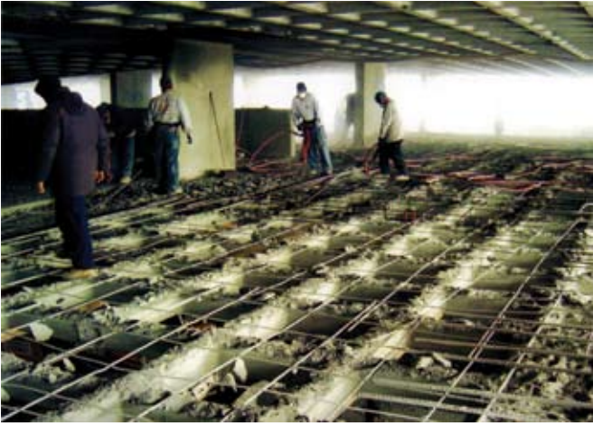
Demolition of a top slab
