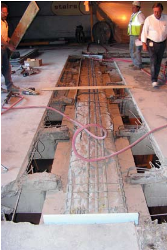
Preparation for full-depth replacement
