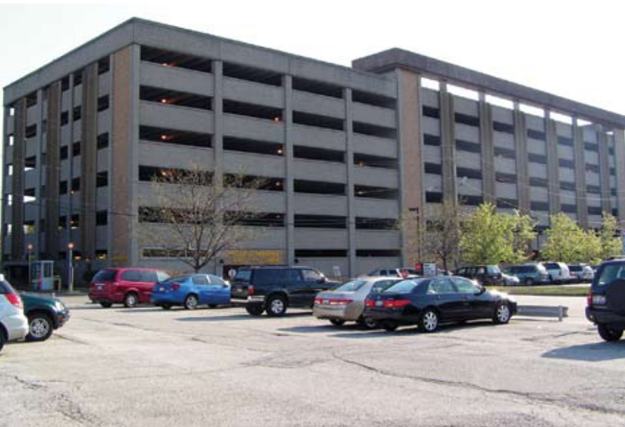
Fairview Hospital Parking Garage
