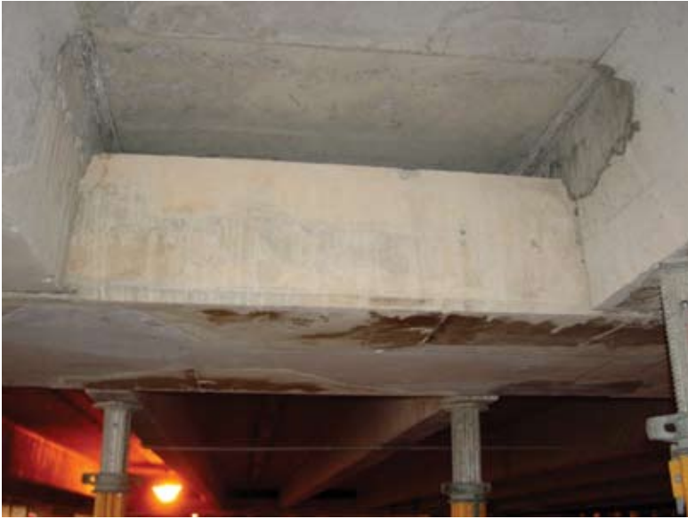
Underside of finished deck repair
