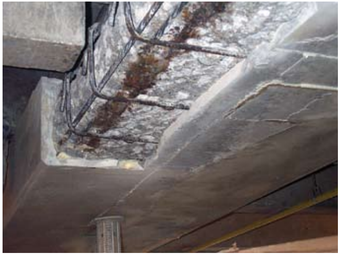
Deck surface preparation, and in some areas, full-depth repair Surface preparation of a beam
