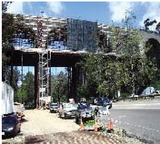
Fig. 2: The entire underside had a very extensive scaffolding system
