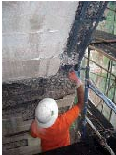
Fig. 3: Cleaned reinforcing steel was coated
