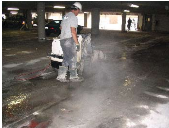
Fig. 1: Sawcutting for slab removal
