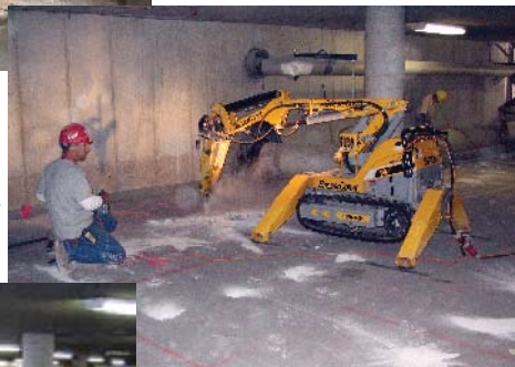
Fig. 3: Demolition robot used for slab demolition and removal
