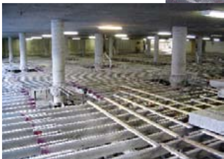
Fig. 4: Unique shoring systems were used on the project
