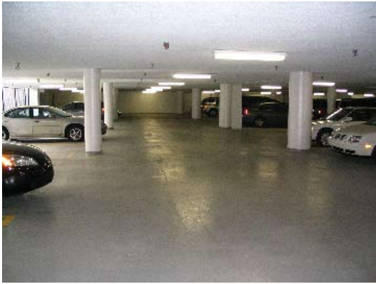
Fig. 5: Finished slab with deck coating
