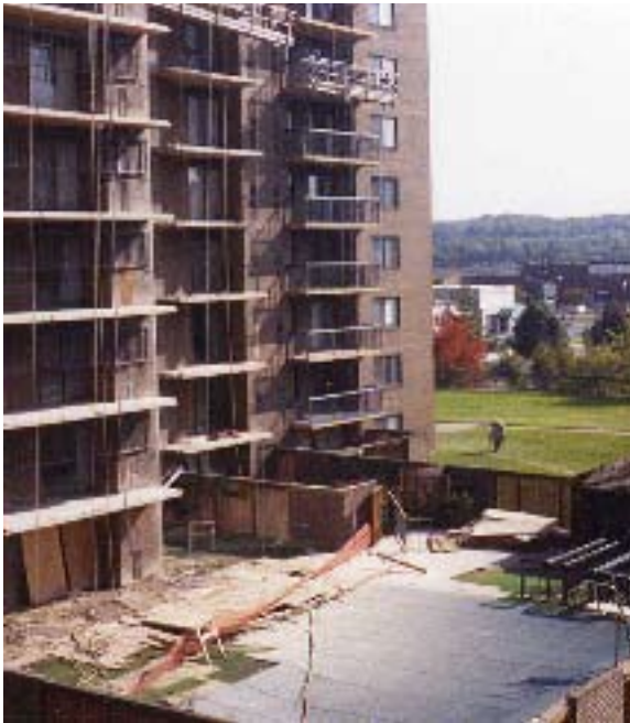
Fig. 3: Phase II work being performed
