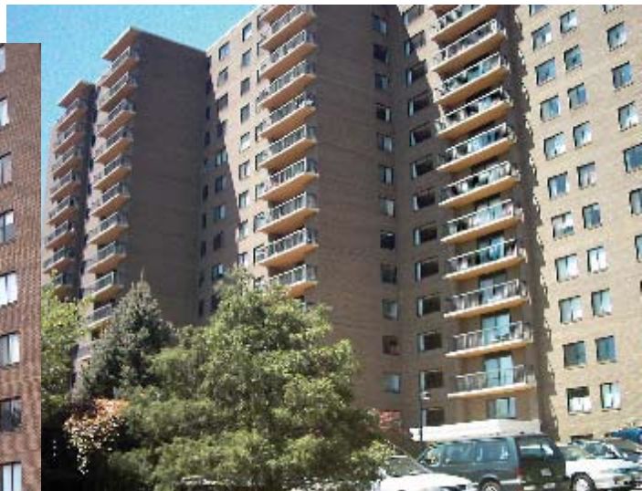
Fig. 2: Phase II work completed in 1991
