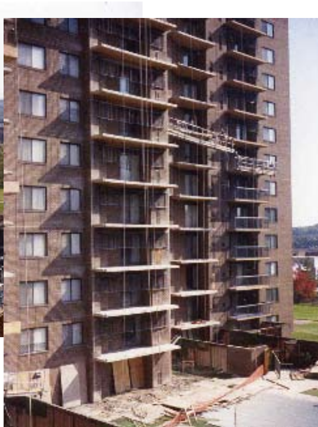
Fig. 4: Phase II work showing swing stage
