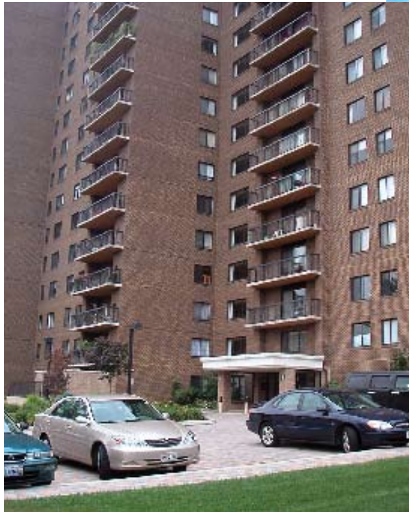
Fig. 1: Repair work done in 1991 has held up very well for 15 years
