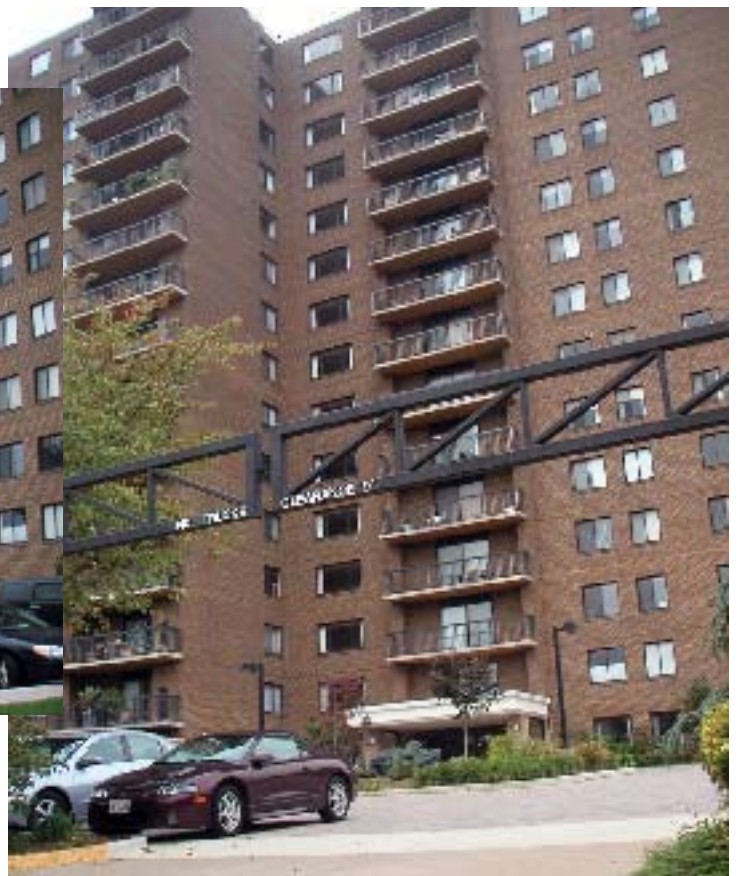
Fig. 6: Another shot of the balconies 15 years later
