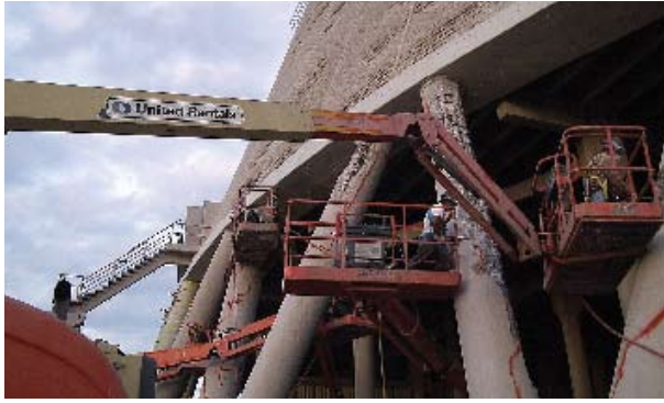
Fig. 3: Delaminated concrete removed with pneumatic chipping guns
