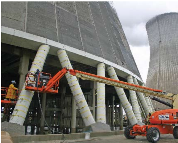
Fig. 1: St. Johns River Power Park Unit No. 2 Hyperbolic Cooling Tower
