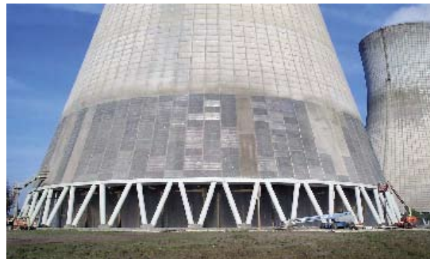
Fig. 6: Finished work on 120 lintel beams and 240 column jackets
