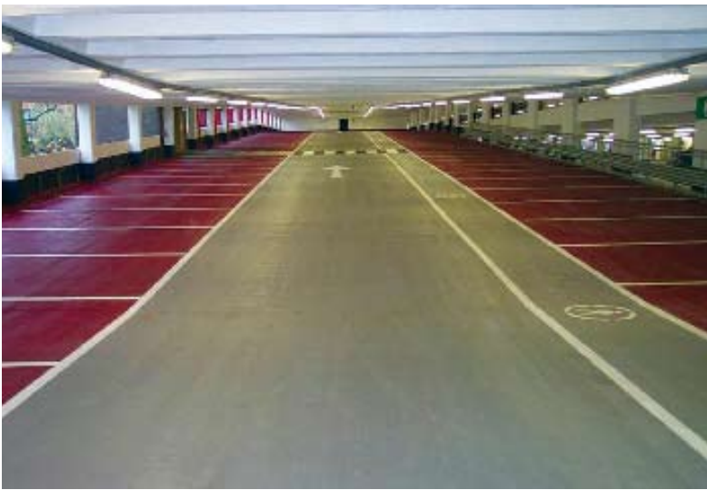
Internal appearance before (top) and after (bottom) refurbishment
