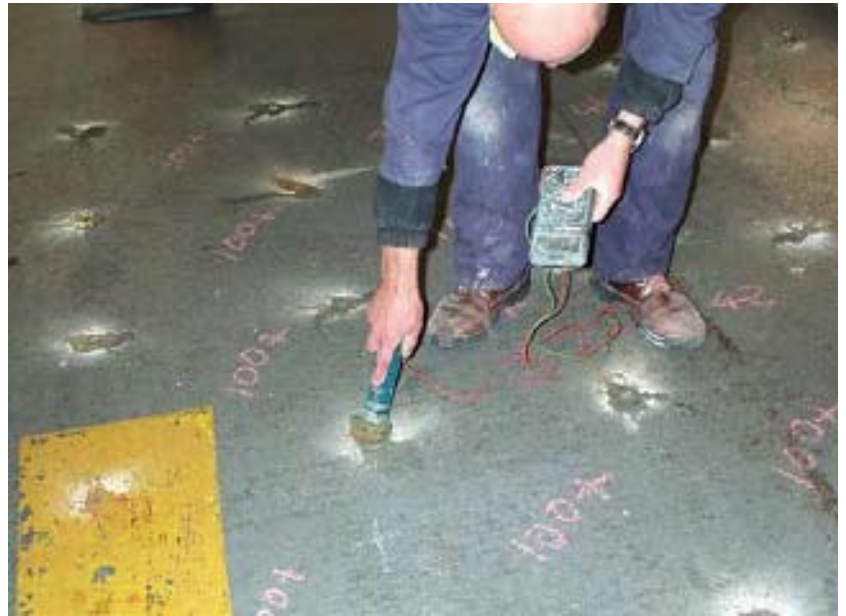
Inspection and evaluation of the structure
