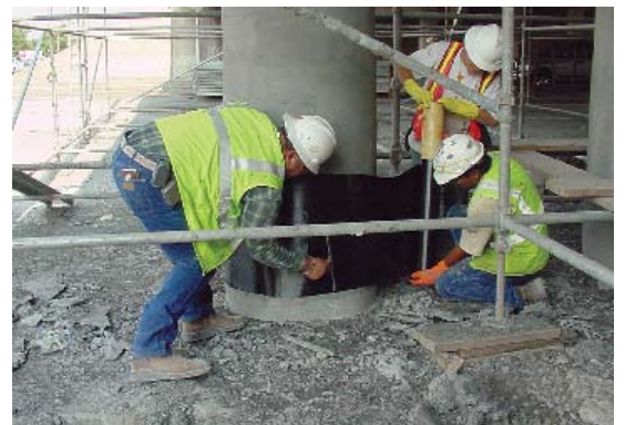
Fig. 4: Installation of CRFP to Column 10
