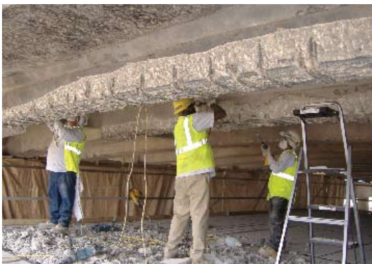
Fig. 3: Removal of delaminated concrete along the beams and deck
