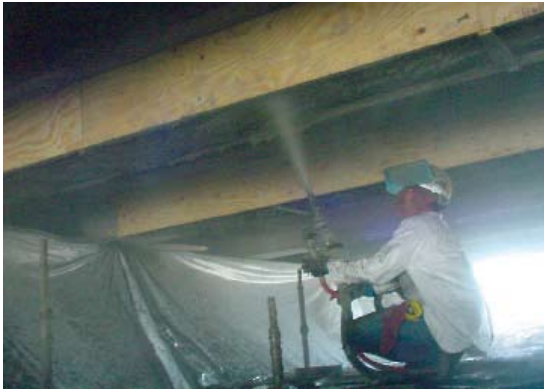
Fig. 5: Wet-spray shotcrete applied to underside of beam
