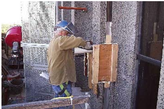
Fig. 3: Placing concrete into formed repair location
