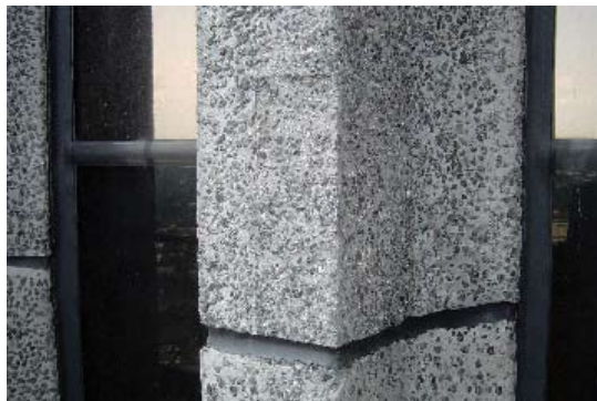
Fig. 6: Completed repair profile—a beautifully exposed garnet aggregate finish
