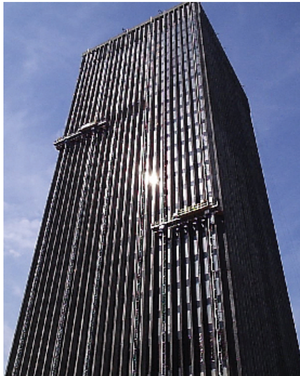
Fig. 1: Repairs took place high above the downtown Rochester, NY, area
