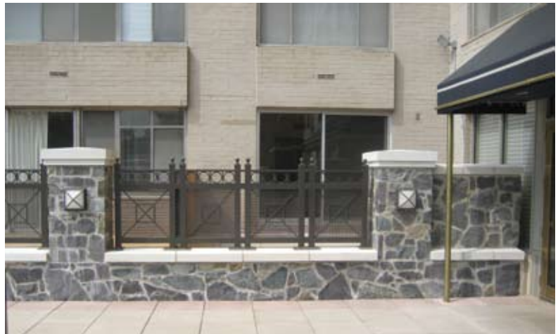
New stone masonry terrace with custom aluminum railing, stone coping, and new lights
