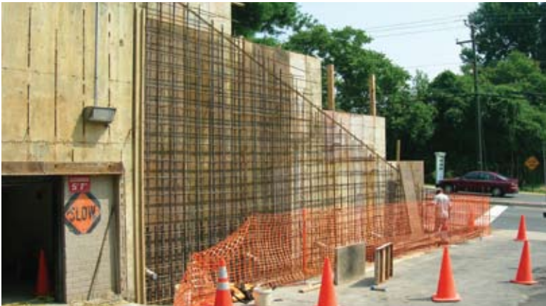
Steel reinforcement for the new driveway retaining wall
