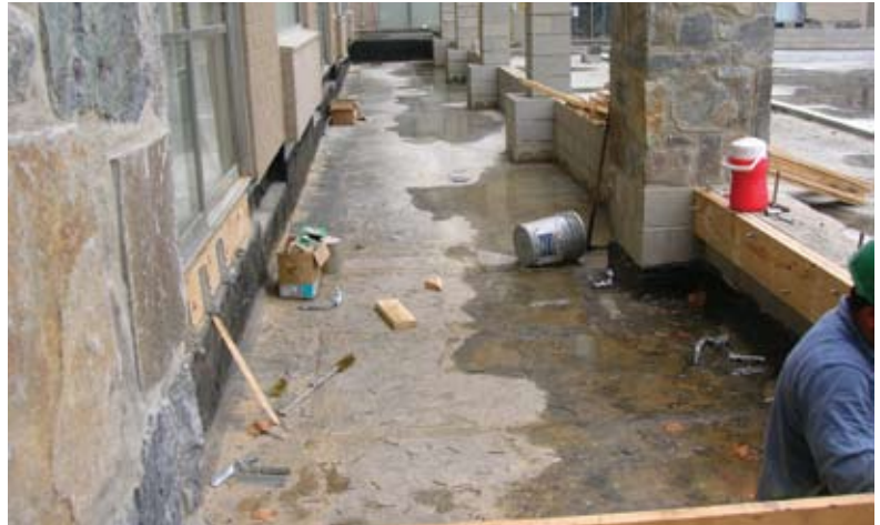
Construction of the terraces
