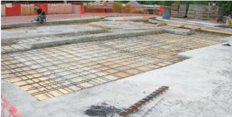
South plaza deck concrete repairs
