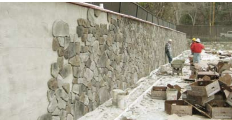
Installing synthetic stone at the pool retaining wall
