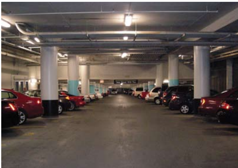
The parking garage after rehabilitation
