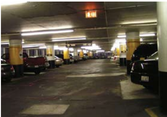
The parking garage before rehabilitation
