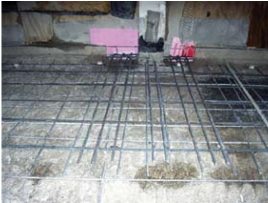
Tapering of slab to resolve punching shear issue
