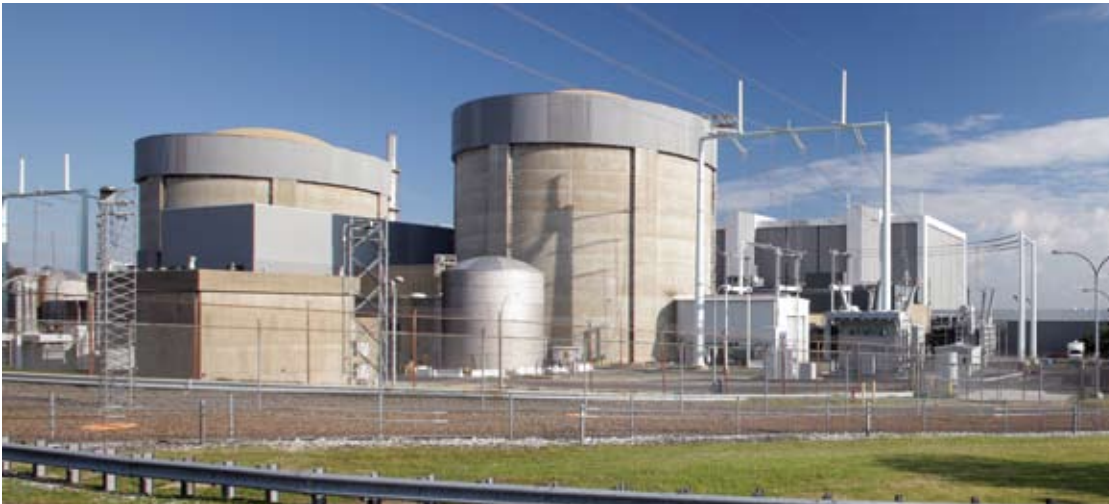
Calvert Cliffs Nuclear Power Plant
