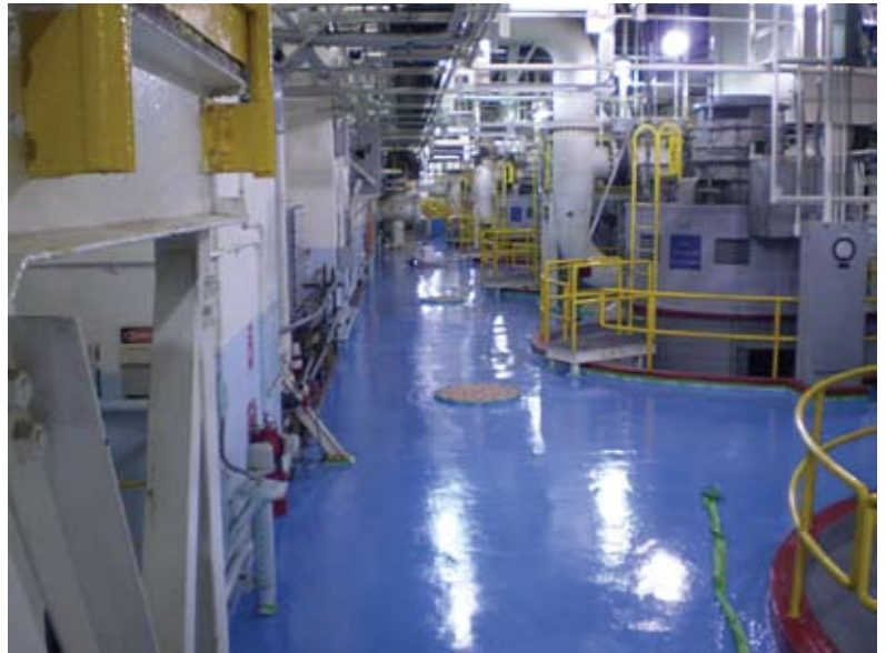
Project completion—Unit 2 of intake structure after floor coatings
