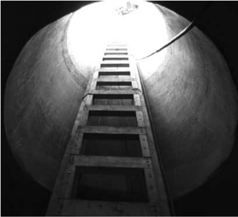
The only access to pipe was through 30 in. (760 mm) diameter manholes
