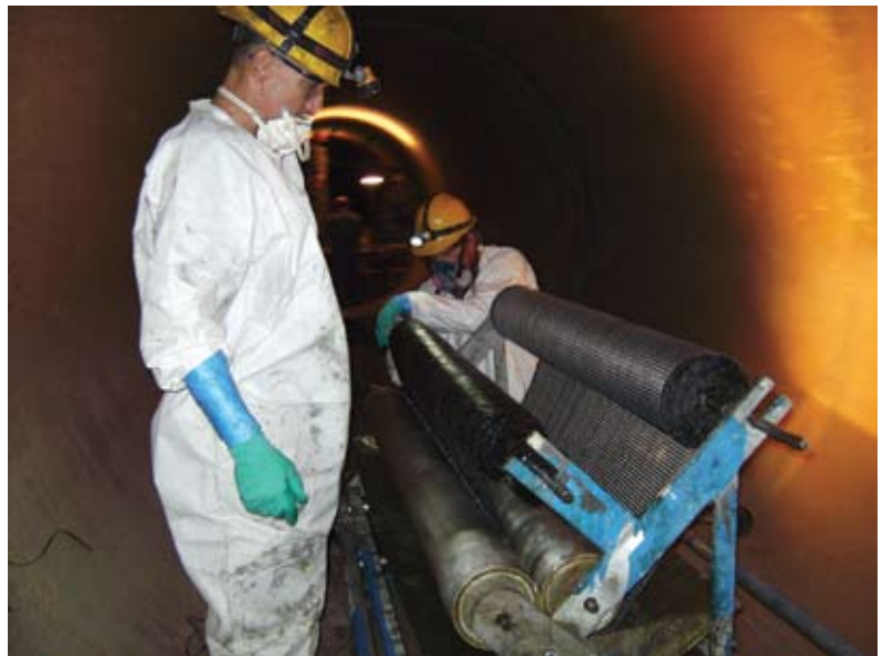
Saturating machine reassembled inside the pipe
