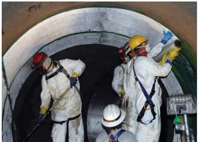
Installation of glass fabric on pipe
