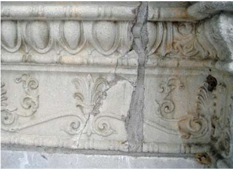
Cast stone on Carrington Hall prior to repairs
