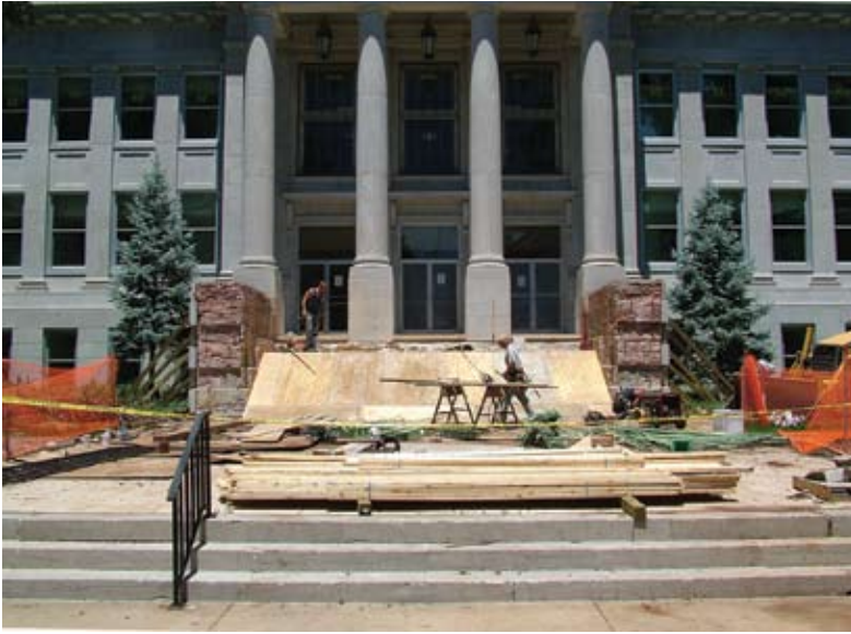
Stair removal and replacement on Sicheluff Hall
