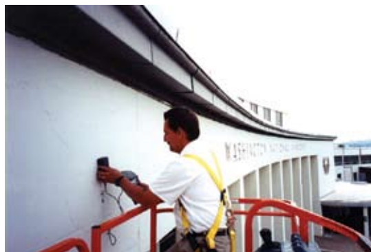
Nondestructive testing was performed including pachometer readings
