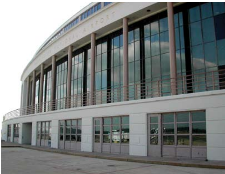
Completion of airside façade
