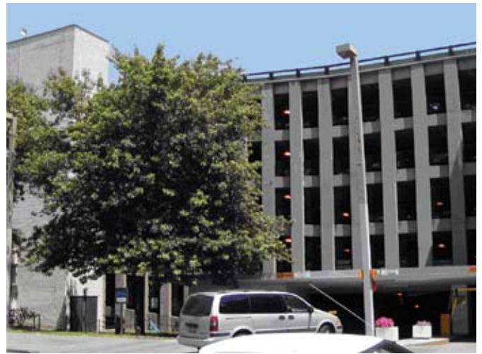
SUNY Health Science Center Brooklyn Parking Structure
