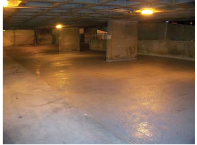
Final surface with vehicular traffic bearing membrane
