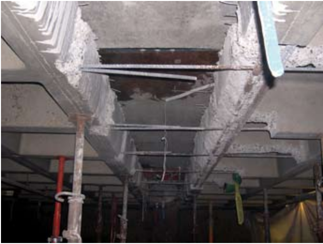
Full-depth concrete repairs
