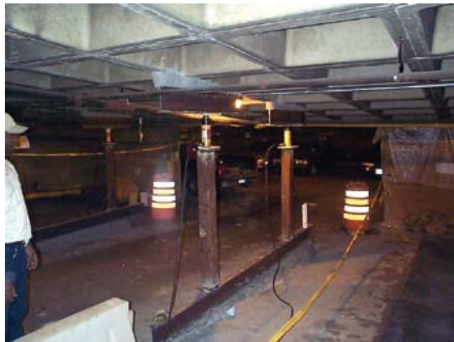
Load test of trial strengthening area
