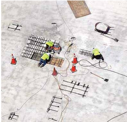
Repairs to top deck prior to waterproofing
