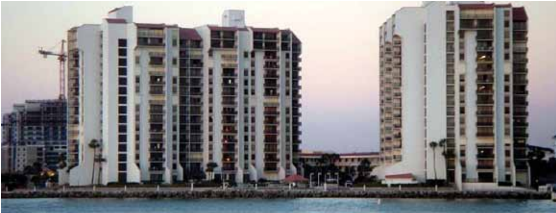
440 West Condominium, "The Concrete Ship." Parking is below grade and below high-tide line
