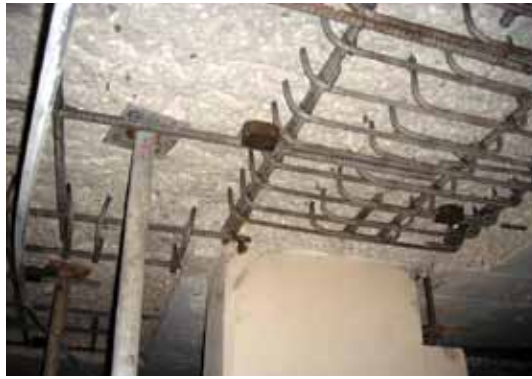
Sacrificial zinc anodes at repair perimeters
